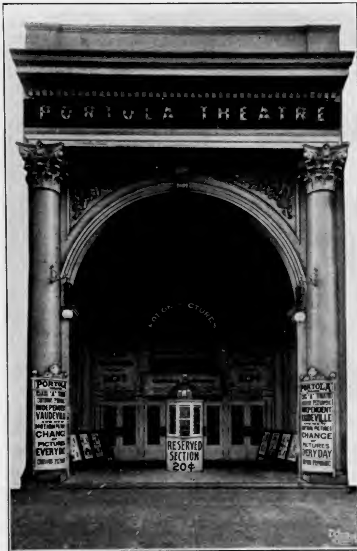
The first fire-proof vaudeville theatre which opened in the downtown district after the big fire. Alberman and Leahy are proprietors and managers playing "Independent" vaudeville. The house opened in April, 1909, with a seating capacity of 1,000. It is situated on Market street, between Third and Fourth, right in the heart of the city.
