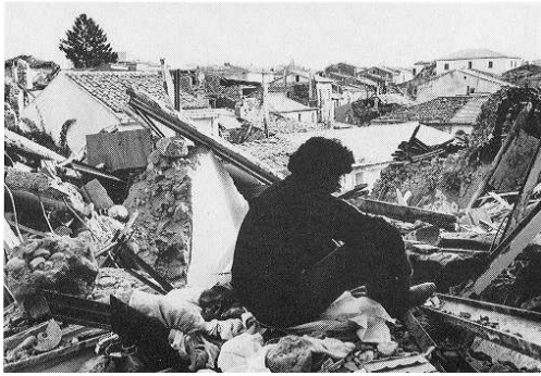
2. After the earthquake.
