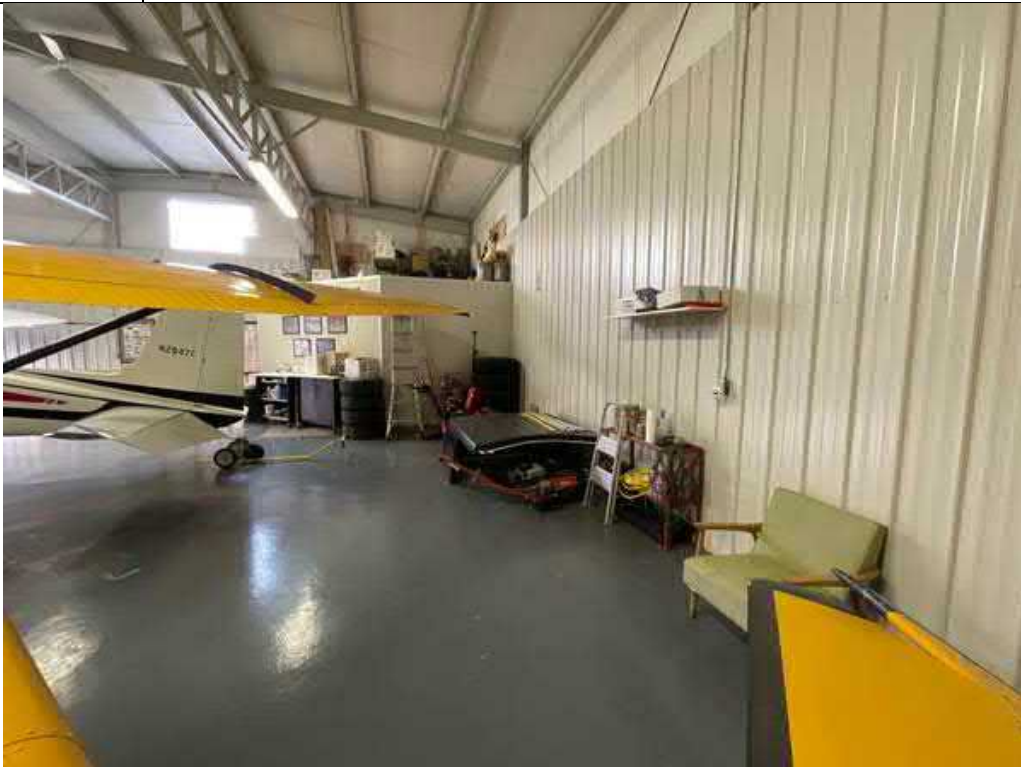
Description Unit 1 - west wall storage Viewing Location/Direction Facing south
