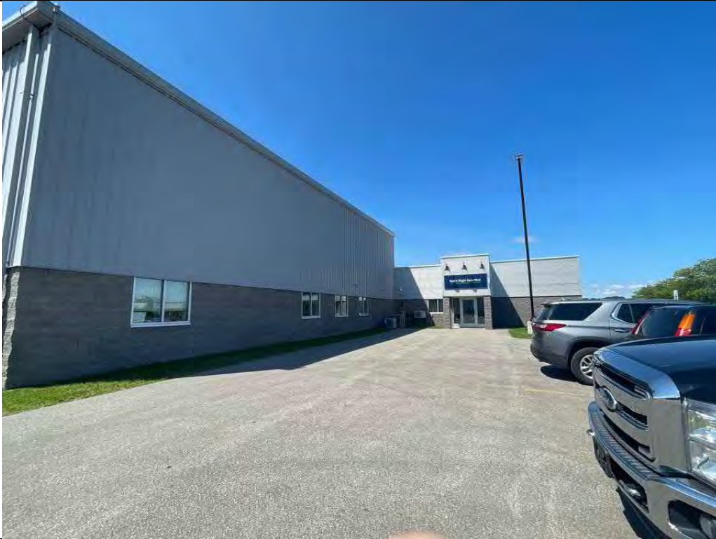
Description South side of east hangar and office entrance Viewing Location/Direction West
