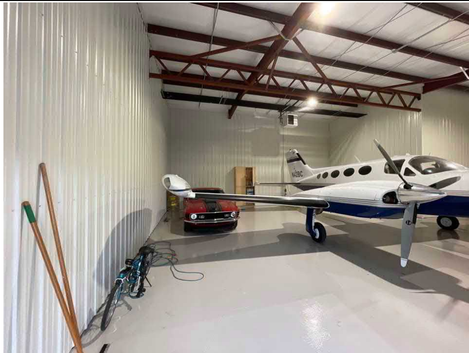
Description Unit 6 Viewing Location/Direction South door facing north
