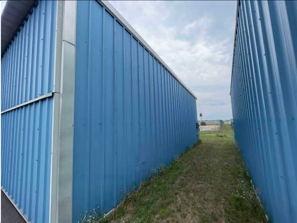
Description South side of building Viewing Location/Direction Facing northeast
