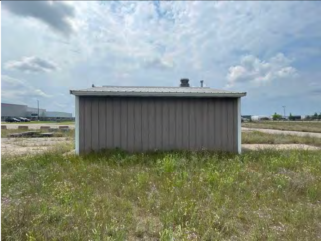
Description East side of building Viewing Location/Direction West
