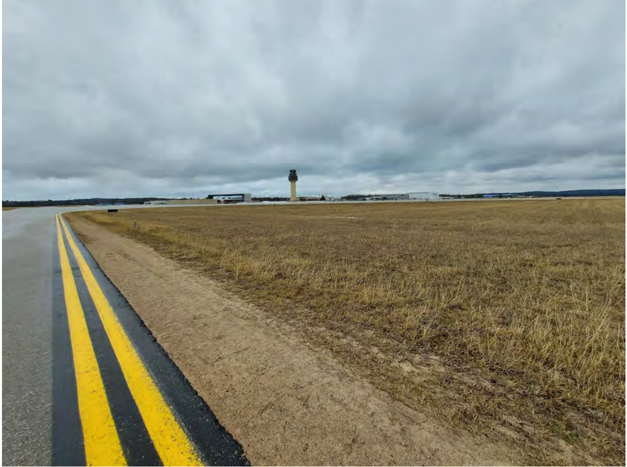
Northeast Corner Taxiways C/D – Future Removal Portion of Taxiway C
