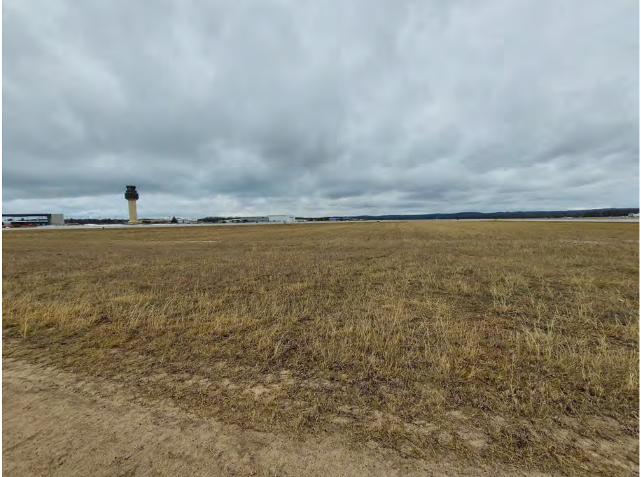
Northeast Corner Taxiways C/D – Future ILS Antenna
