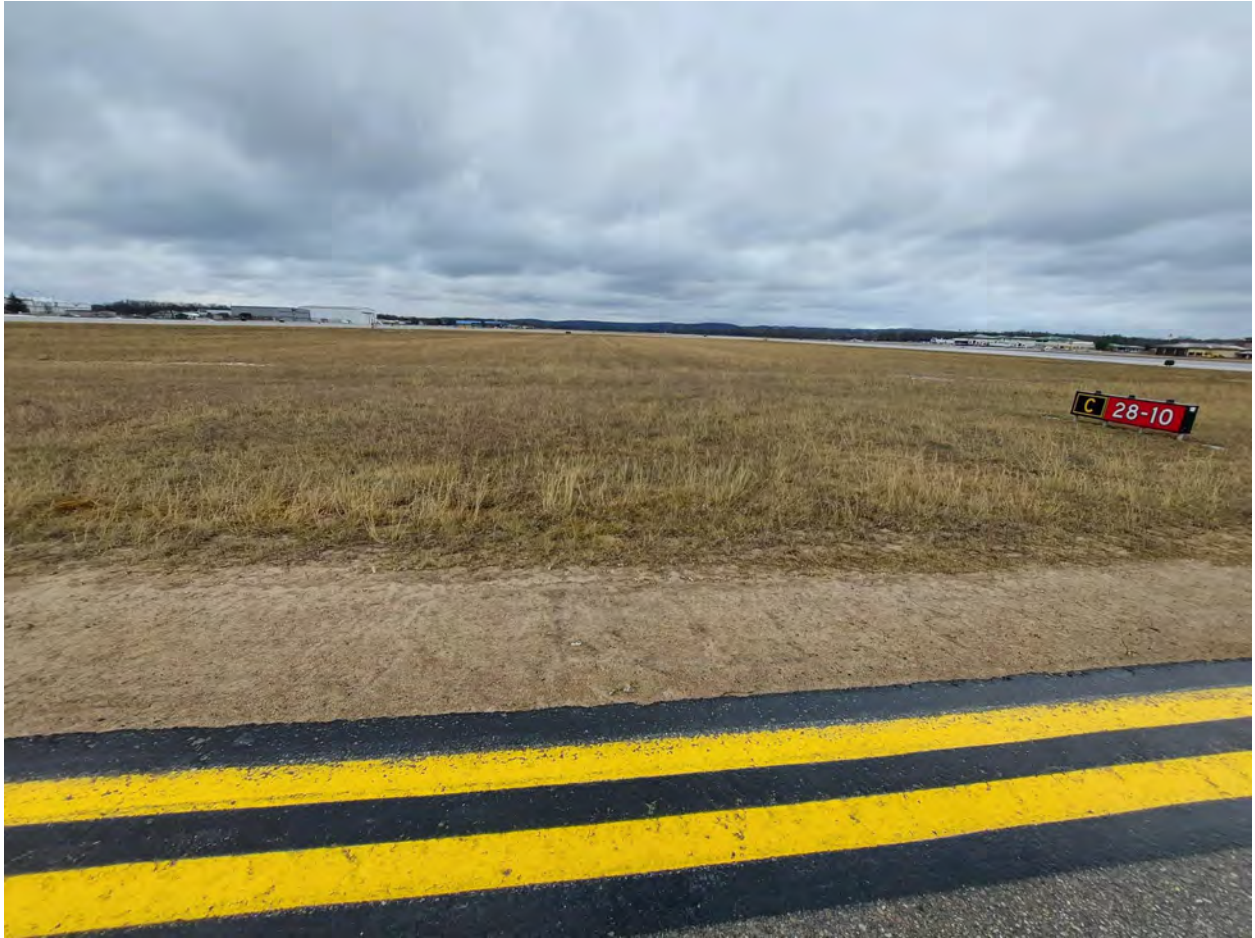
Northeast Corner Taxiways C/D – Future ILS Antenna
