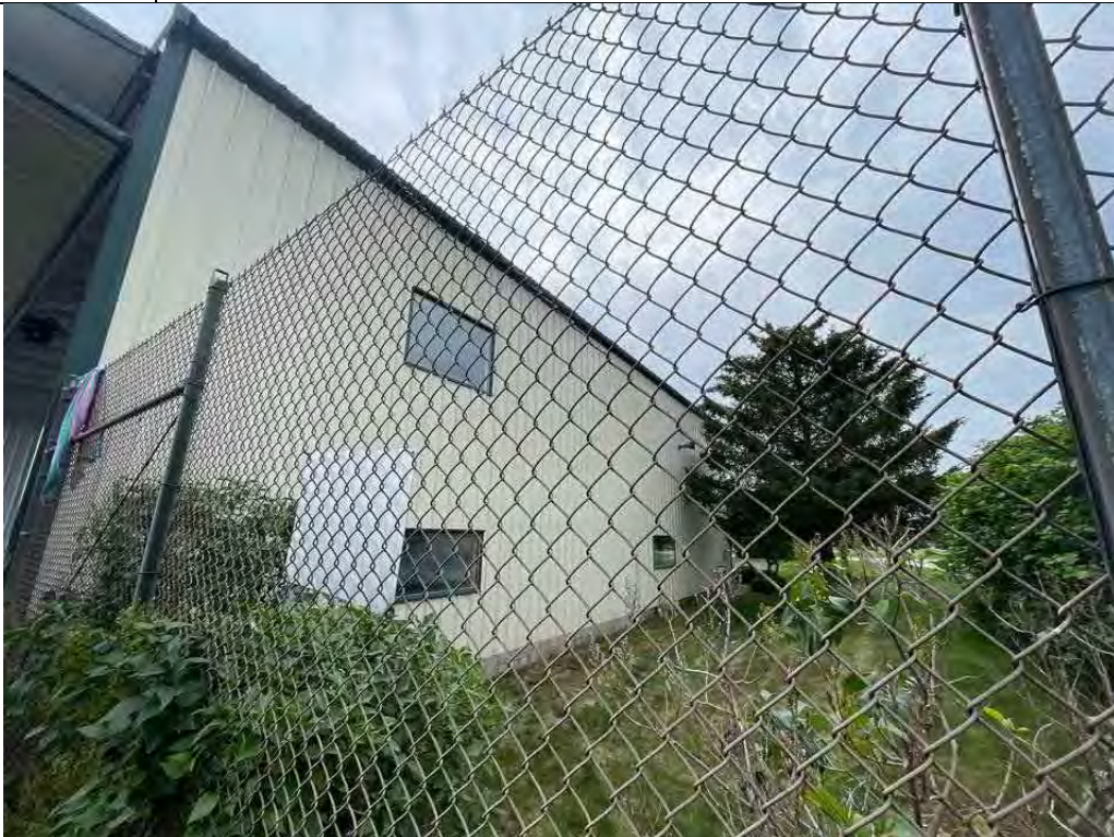
Description South side of building Viewing Location/Direction Northeast
