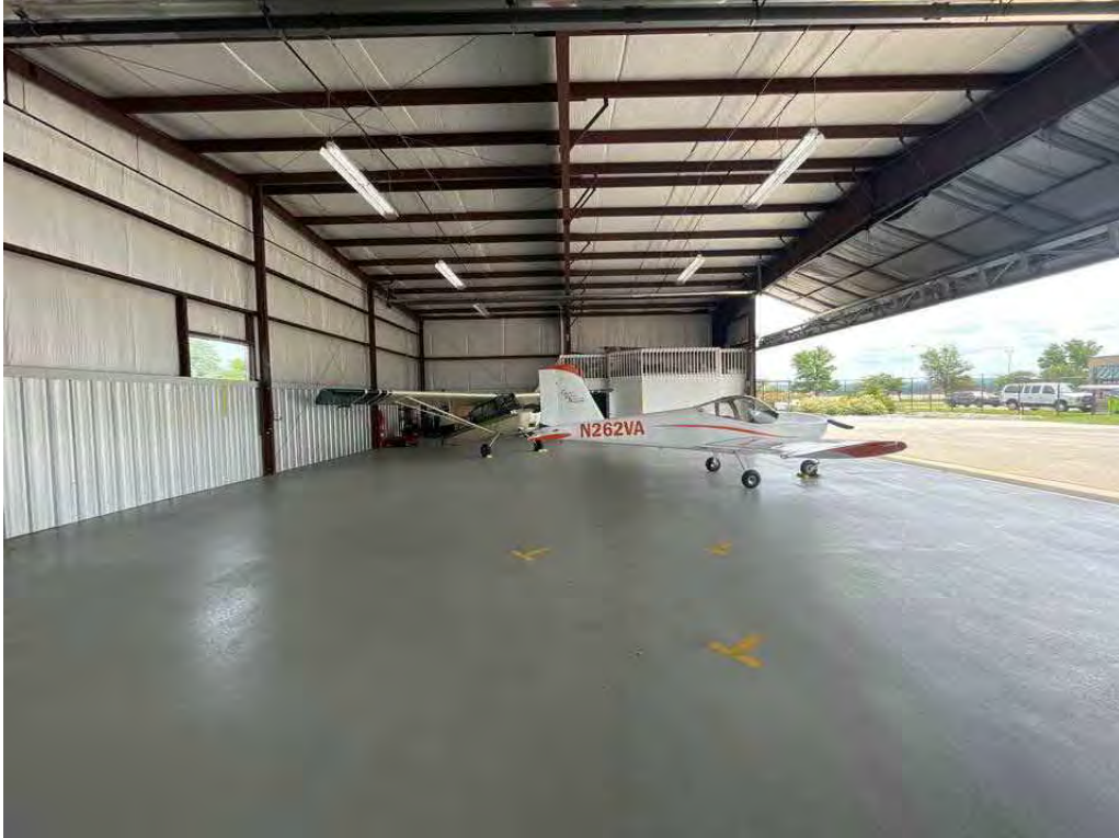
Description West hangar interior Viewing Location/Direction West wall facing east
