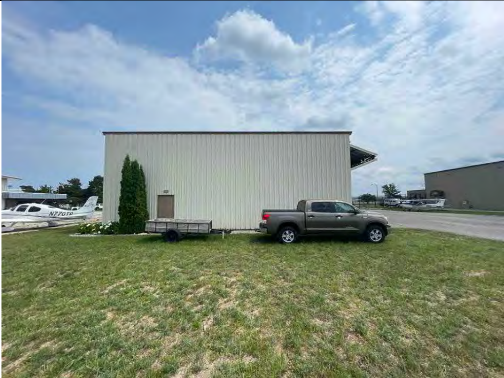
Description West side of building Viewing Location/Direction Facing east
