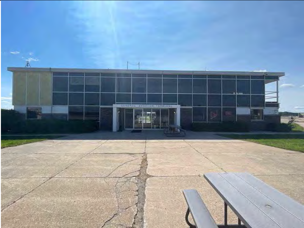
Description Building from west side Viewing Location/Direction East
