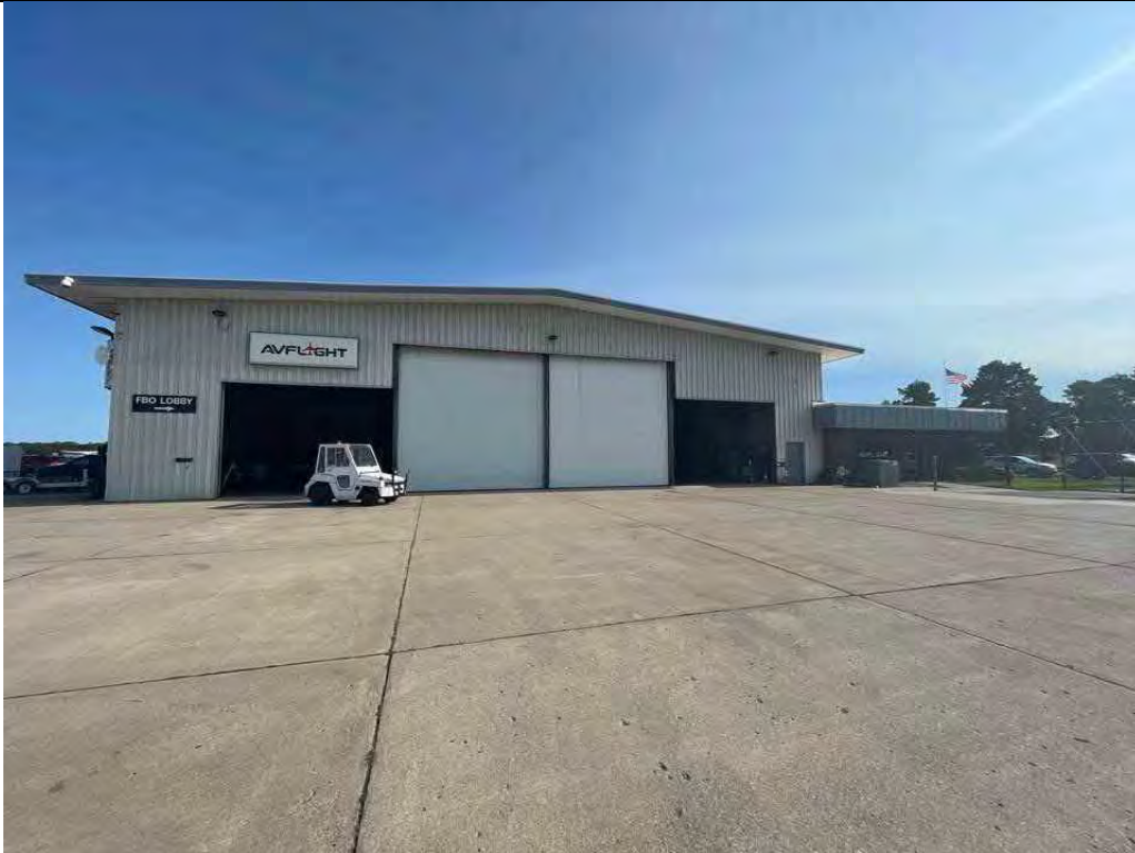
Description South side of building Viewing Location/Direction Facing north
