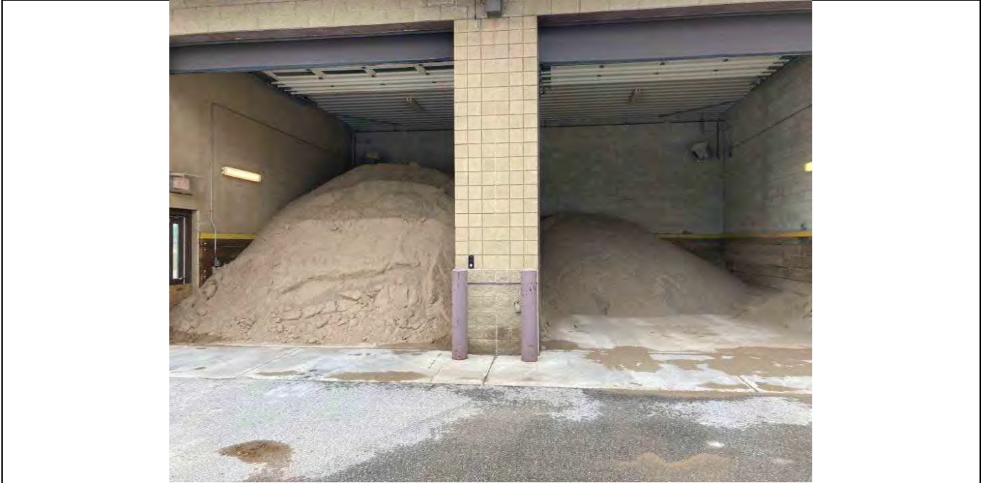
Description Sand storage bays Viewing Location/Direction Looking west
