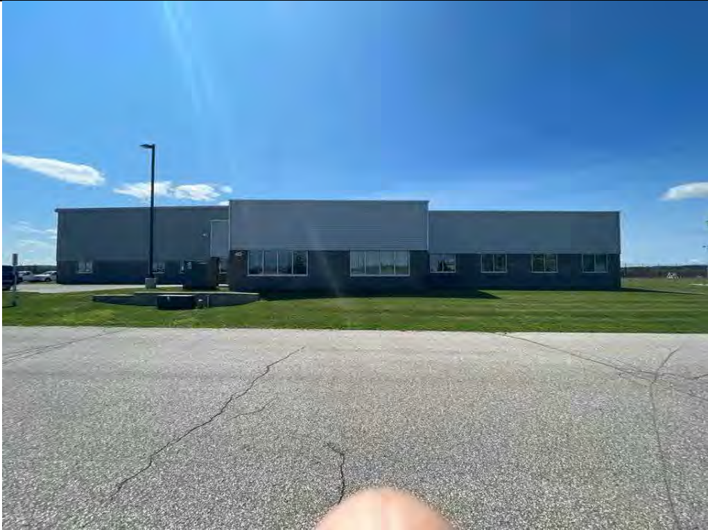
Description North side of building/offices Viewing Location/Direction South
