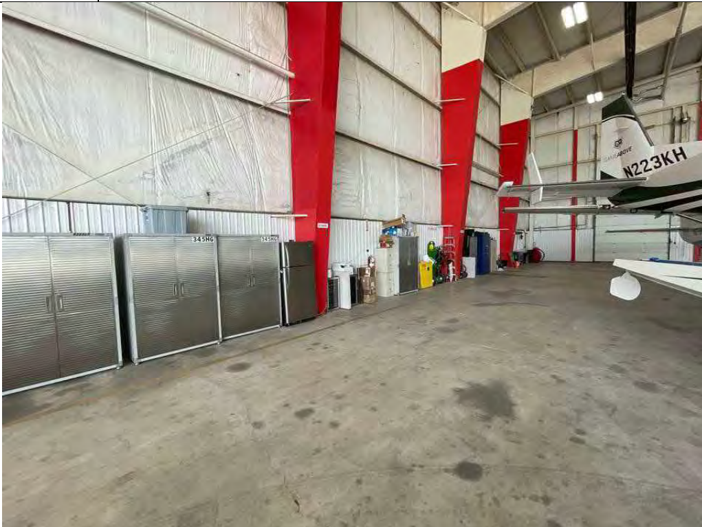
Description West wall storage Viewing Location/Direction West wall facing northwest
