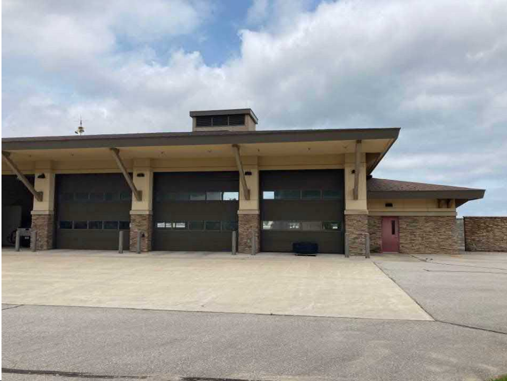
Description South side of fire station Viewing Location/Direction Looking north
