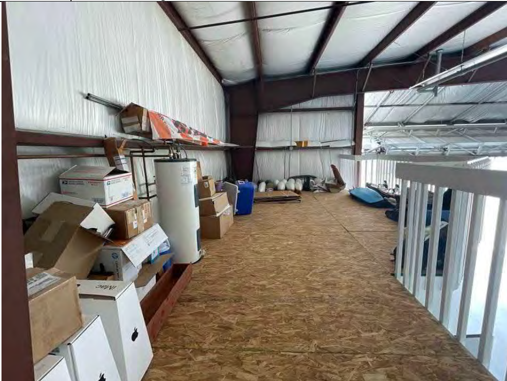
Description West hangar upstairs storage Viewing Location/Direction Facing south
