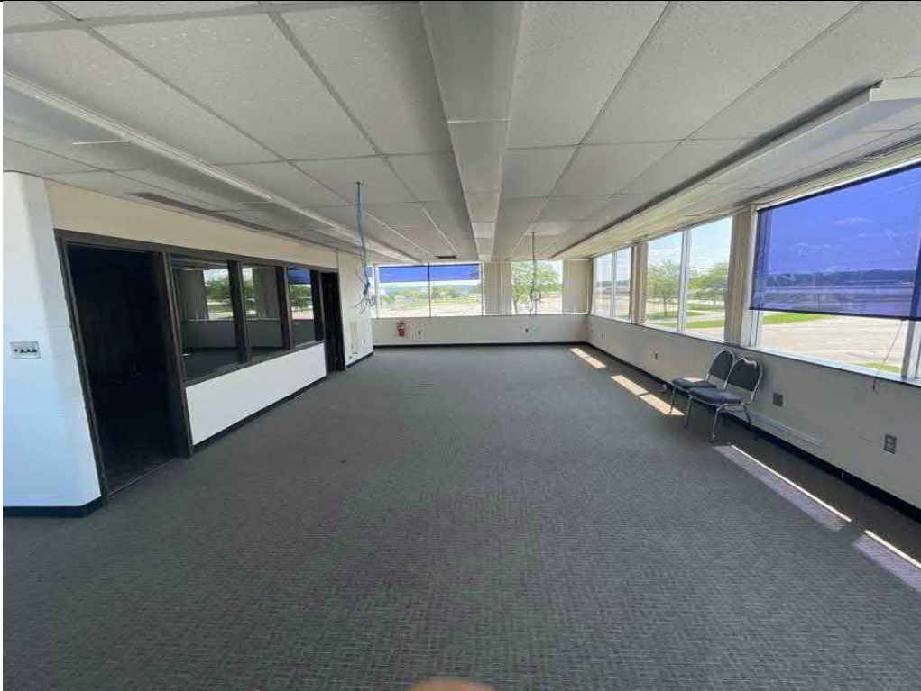
Description South side of upstairs Viewing Location/Direction South building facing east
