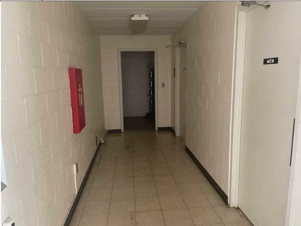
Description North hallways - main floor Viewing Location/Direction North
