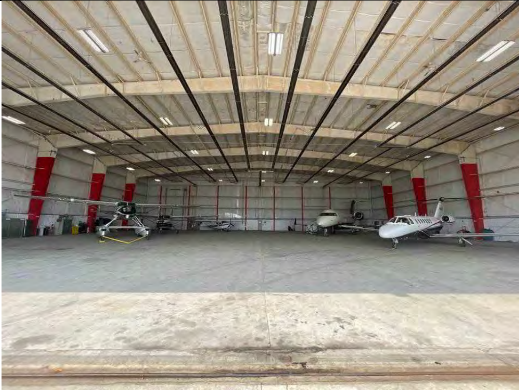
Description Overall interior of hangar Viewing Location/Direction North
