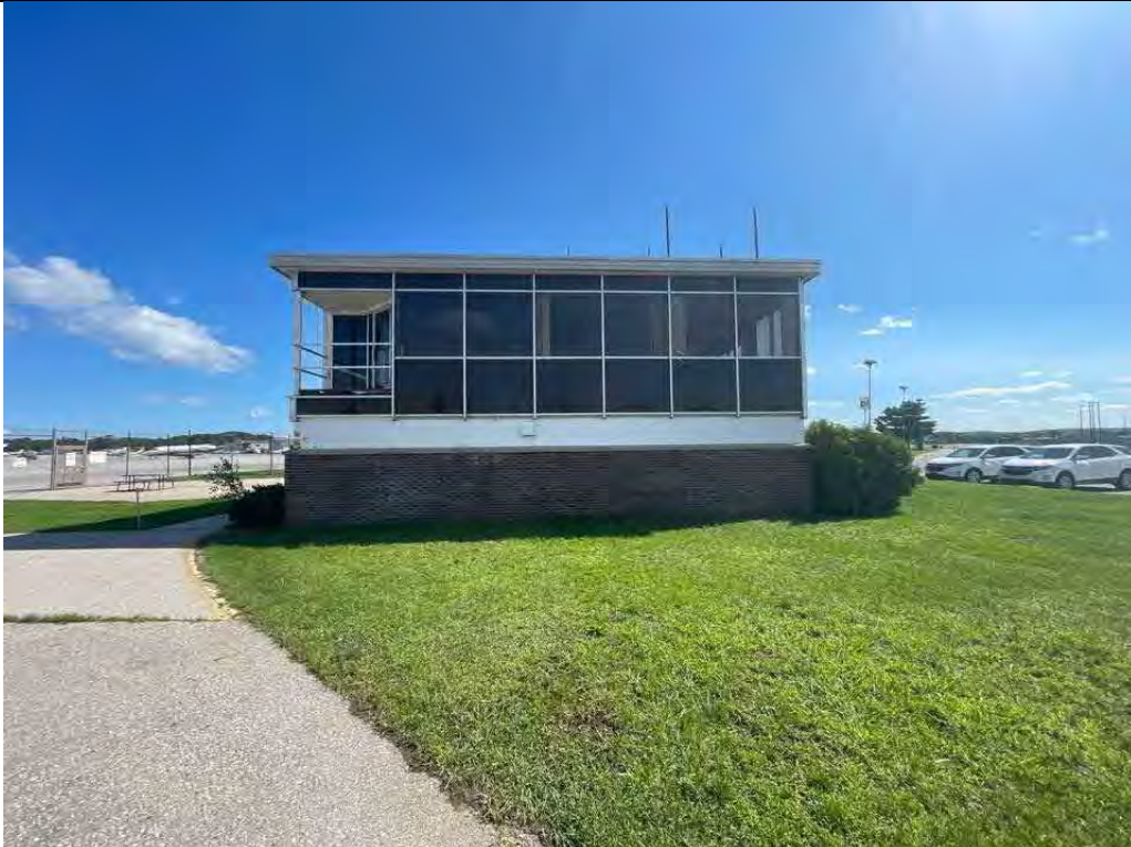
Description South side of building Viewing Location/Direction North
