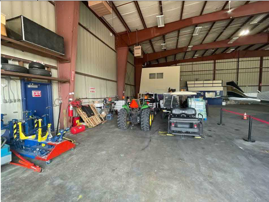
Description West storage area Viewing Location/Direction West building facing north
