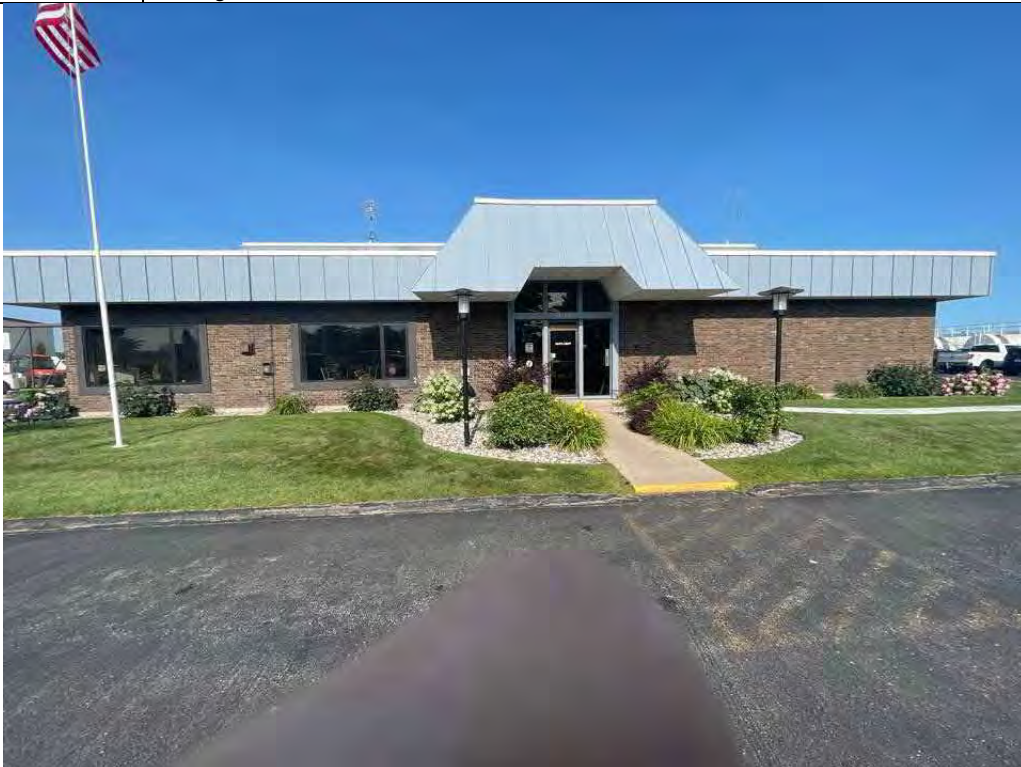
Description Front of building - east side Viewing Location/Direction West
