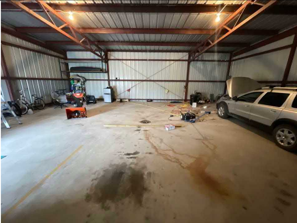
Description Interior overall Viewing Location/Direction Facing west
