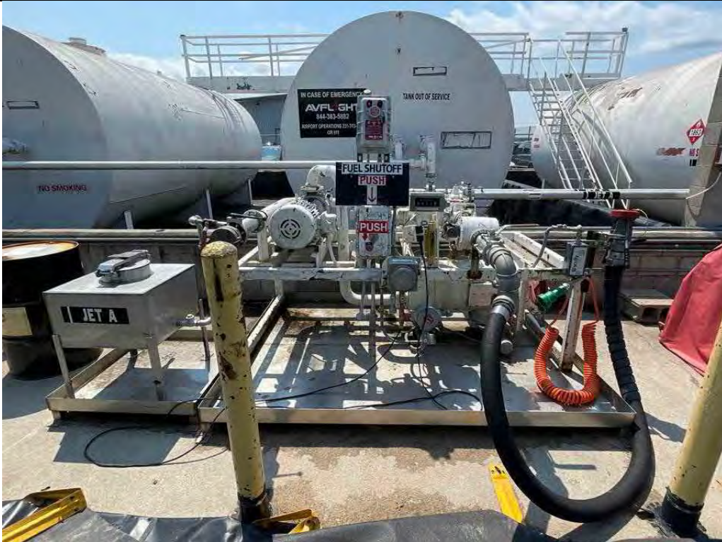
Description Fuel pumps and oil/water separator on left Viewing Location/Direction Facing south
