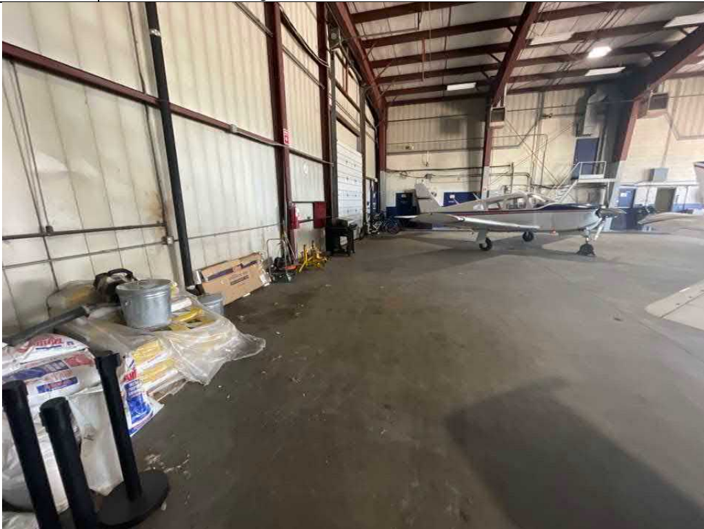
Description North wall storage Viewing Location/Direction North wall facing east
