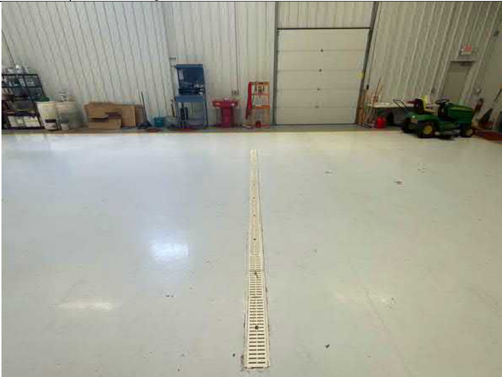
Description Trench drain in south hangar Viewing Location/Direction East
