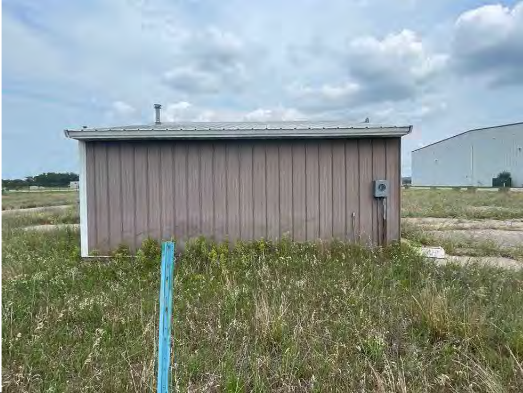
Description West side of building Viewing Location/Direction East
