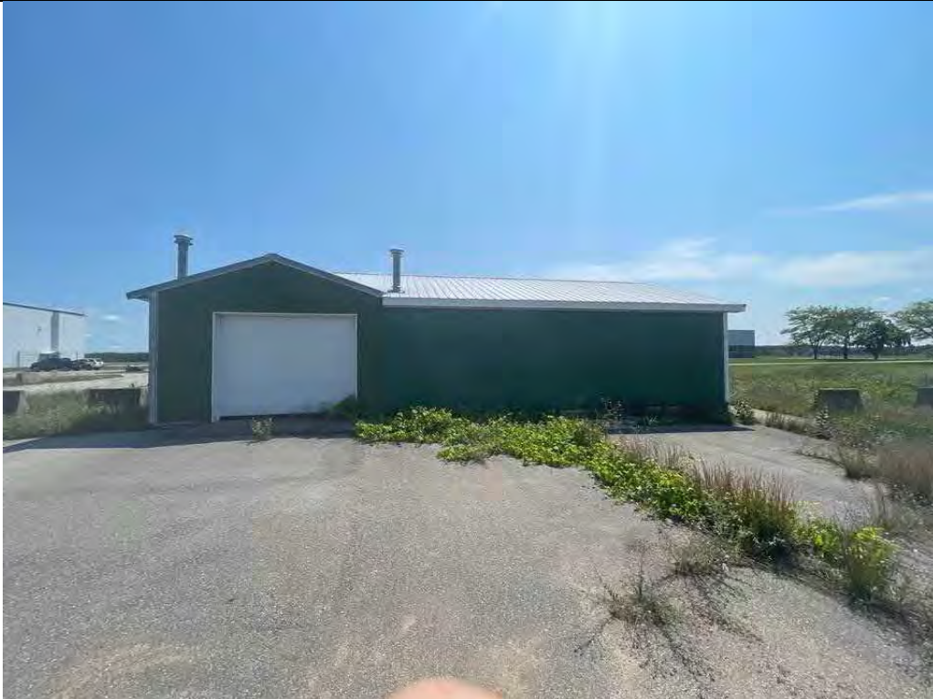
Description North side of building Viewing Location/Direction South
