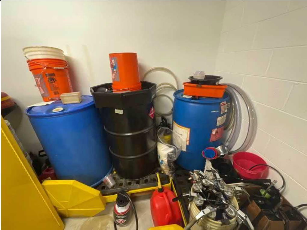
Description Used oil drums and fuel drums Viewing Location/Direction Hazmat storage room
