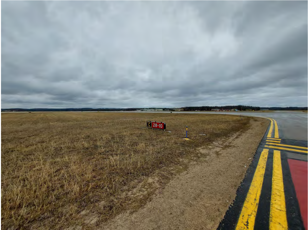
Northeast Corner Taxiways C/D – Future ILS Antenna
