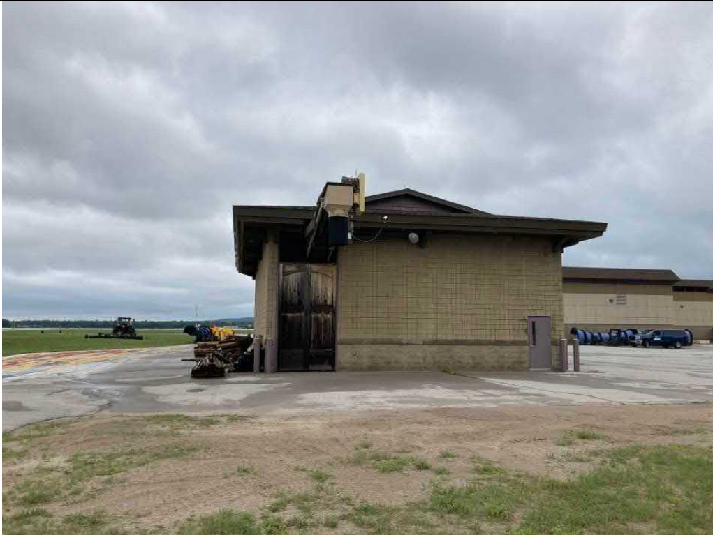
Description South side of sand storage building Viewing Location/Direction Looking north
