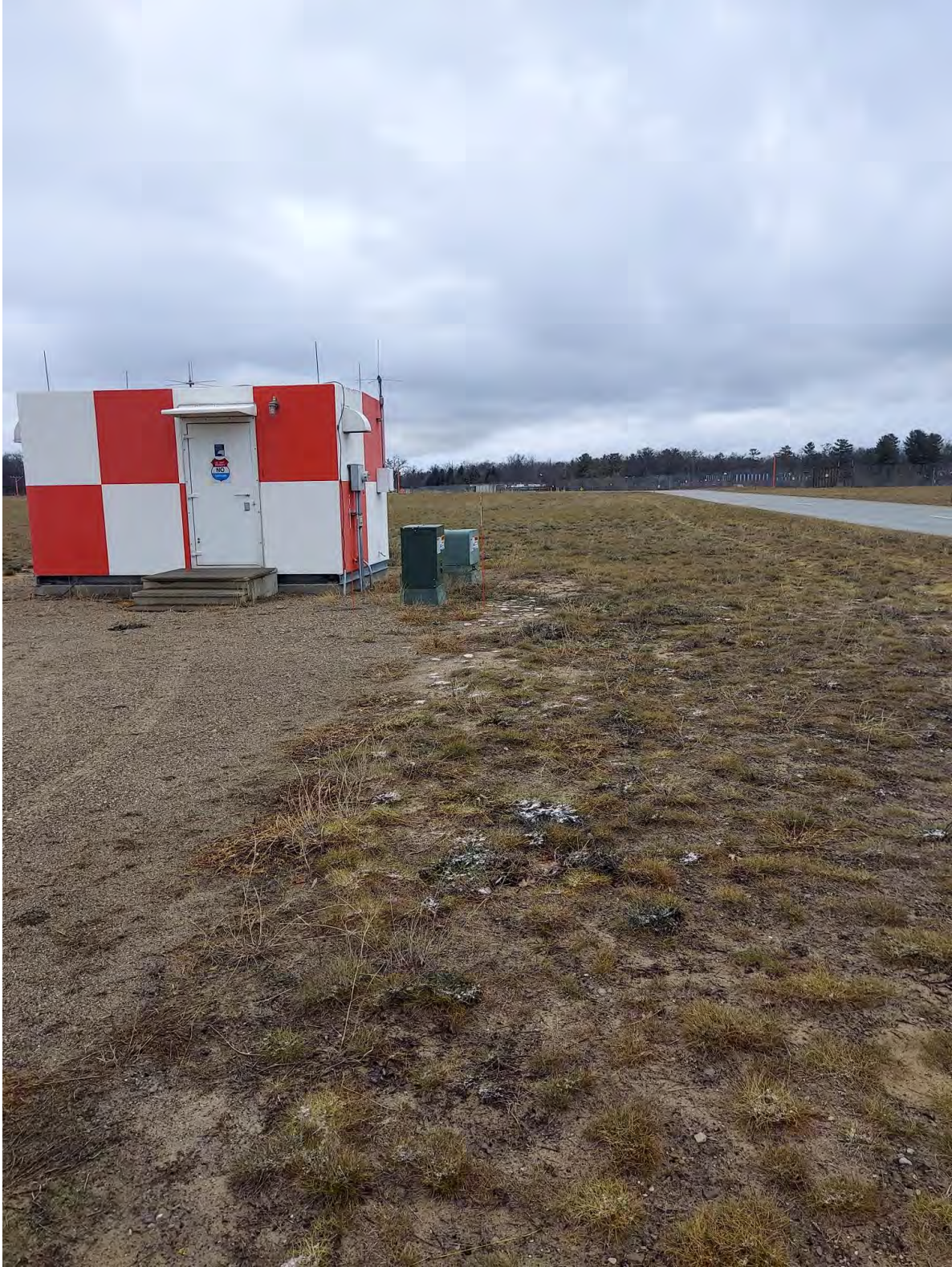
Southeast Runway 28 Threshold – Future Localizer Shelter
