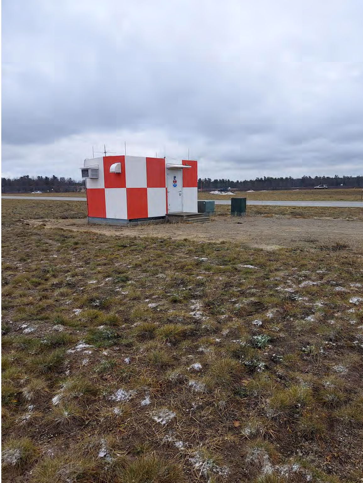
Southeast Runway 28 Threshold – Future Localizer Shelter
