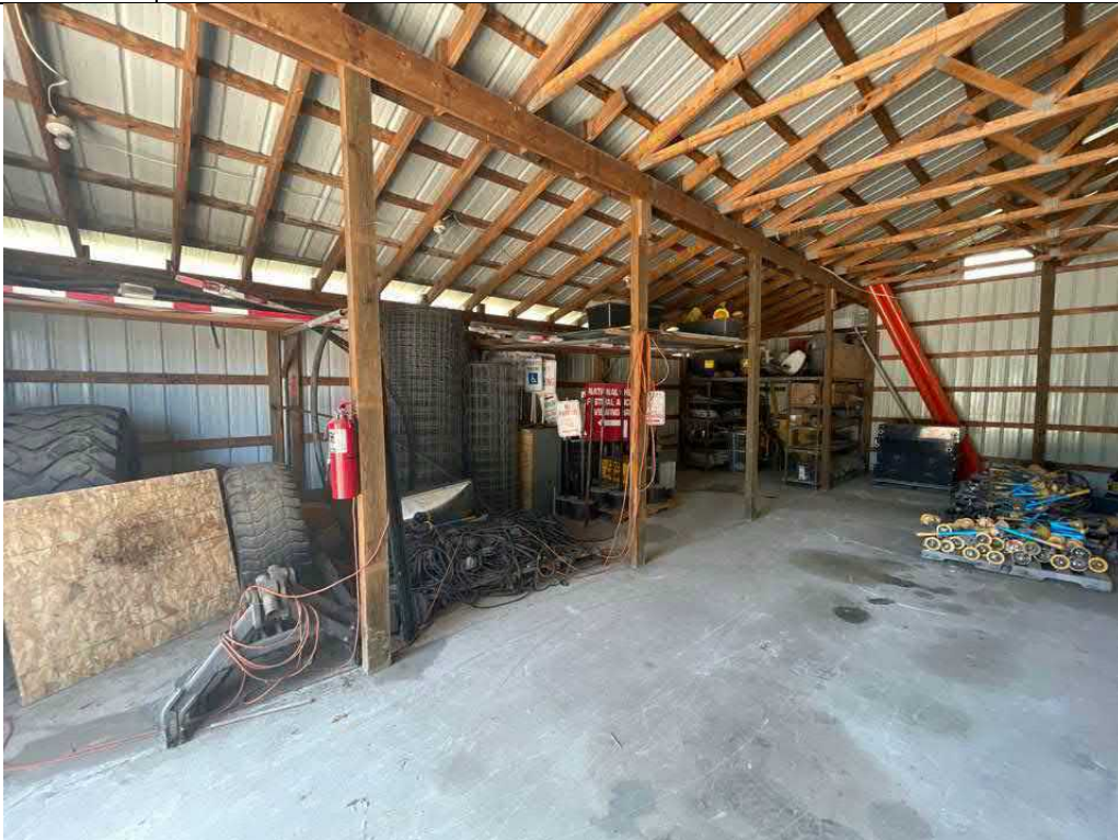
Description South side of storage building Viewing Location/Direction West
