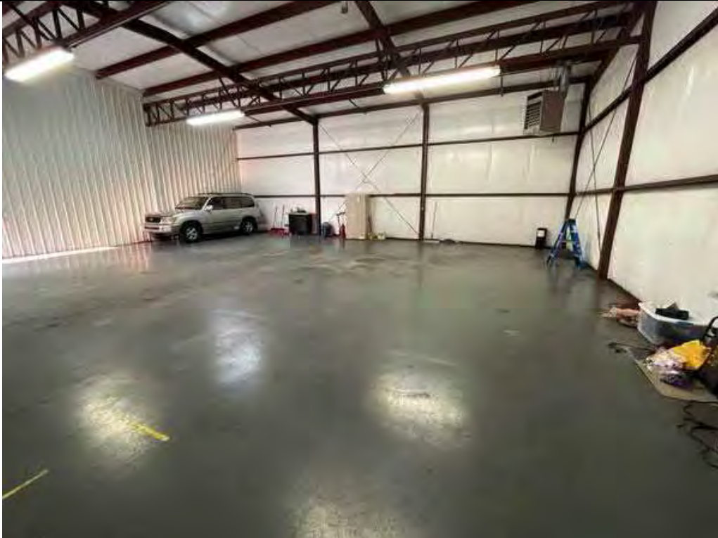
Description Unit 3 interior overall Viewing Location/Direction Facing southwest
