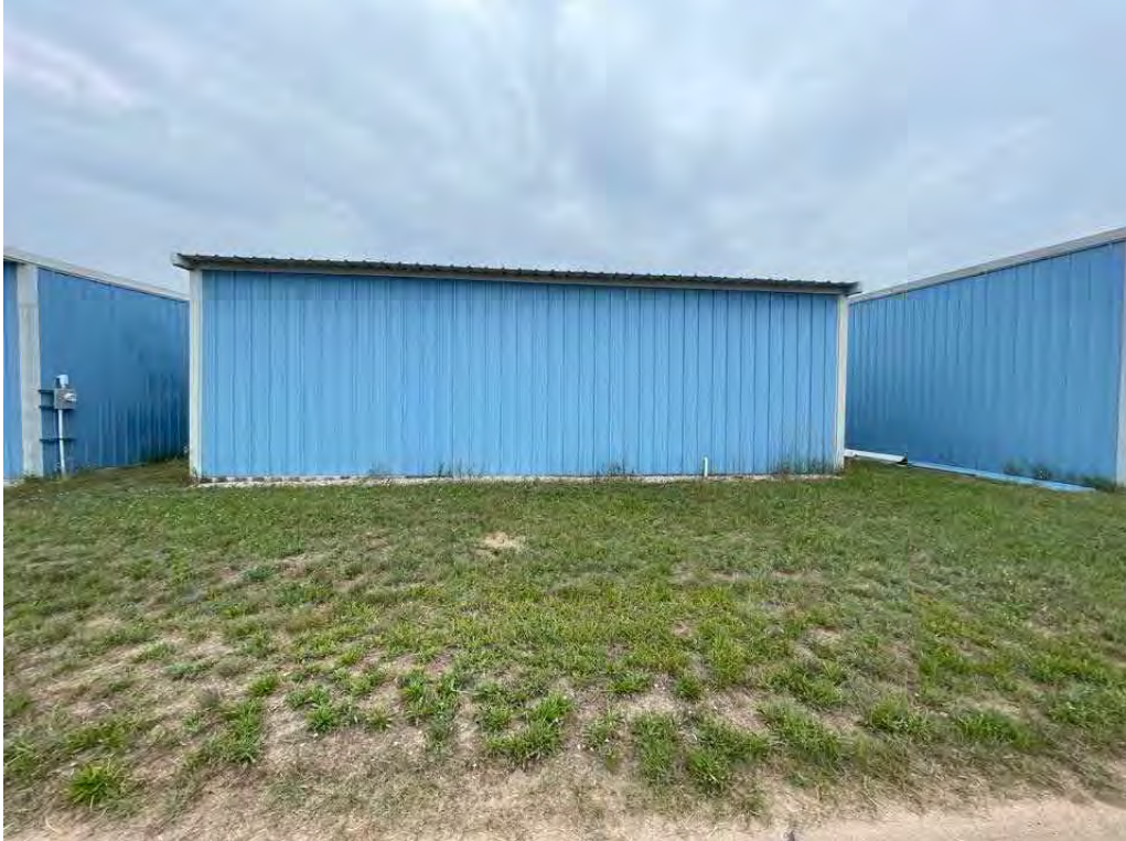
Description East side of building Viewing Location/Direction Facing west
