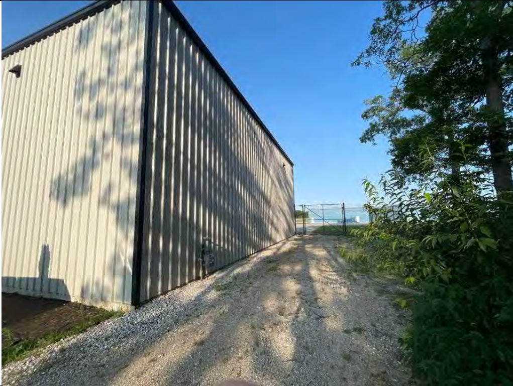
Description North side building Viewing Location/Direction West
