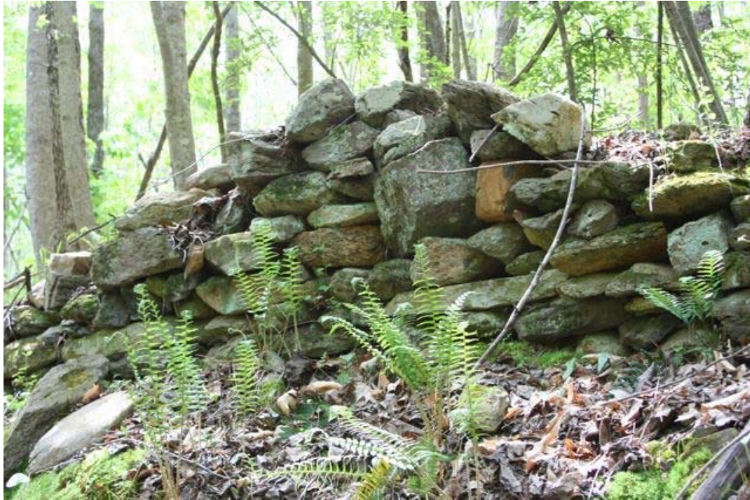
Figure 13: A man-made rock wall structure discovered during the Robeson Creek inventory should be investigated for its historical significance
