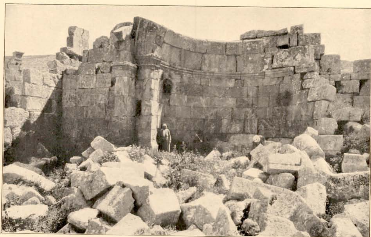
Ill. 221. Qasr il-Benât, Church of Convent. Interior, looking East.
