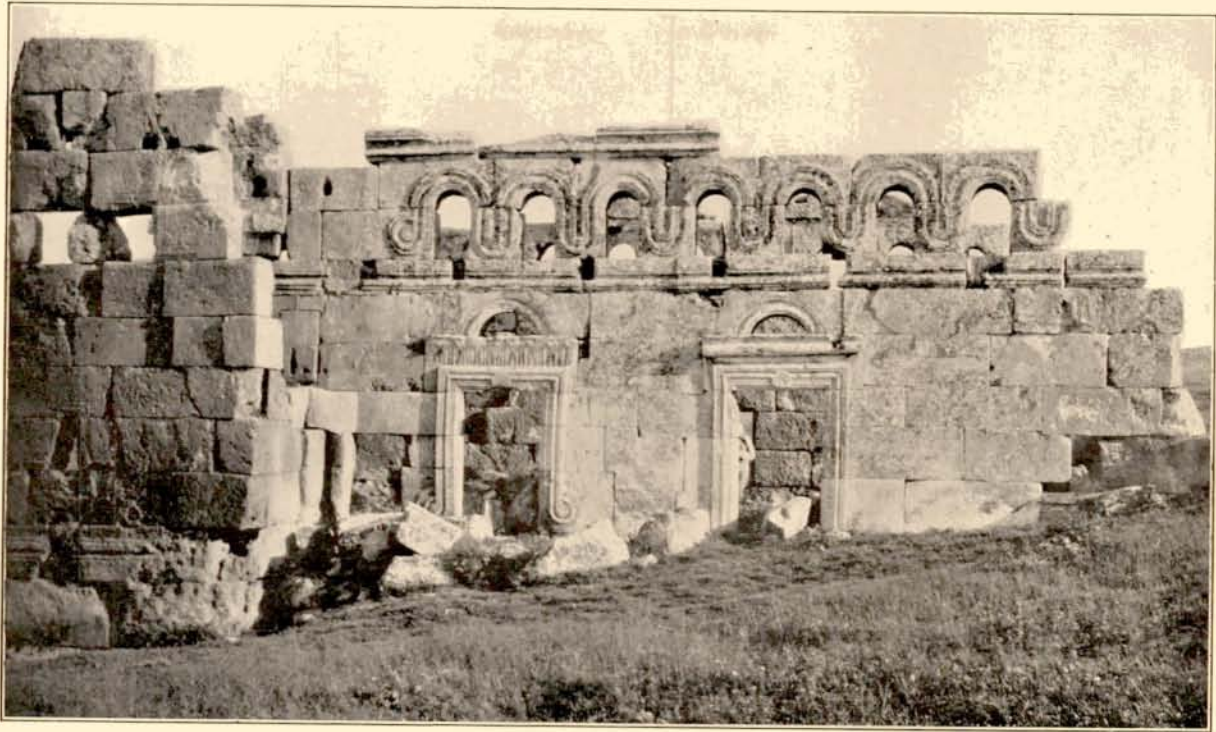
Ill. 226. Kfellüsín, Chapel, North Side.
