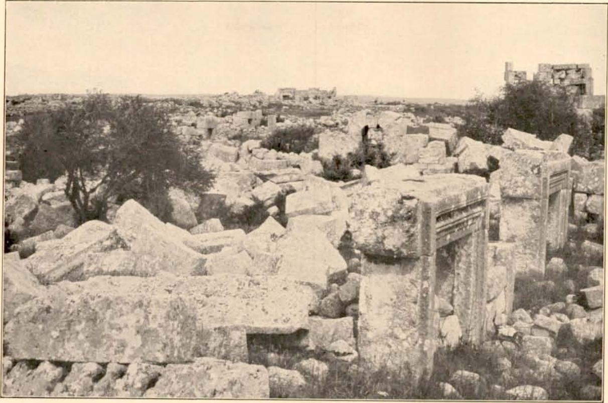
Ill. 261. Fidreh. Ruins of Church. View from the Southwest.
