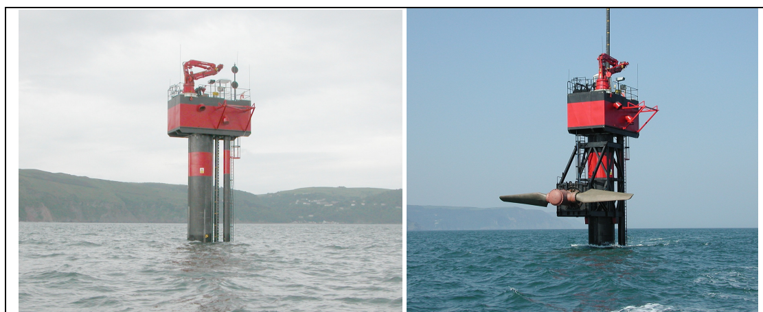
Figure 1.2 Seafloor shown with its rotor submerged (left) and raised out of the water (right)
