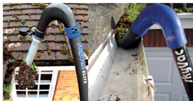
Gutter Cleaning using SkyVac high reach technology
