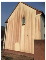
Softwashing to remove green red or black organic matter
