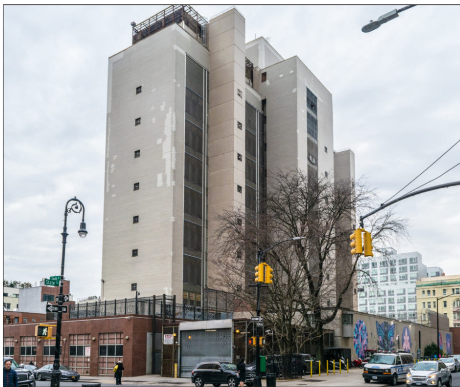
The Brooklyn Detention Complex located on Atlantic Avenue. Eagle file photo by Rob Abruzzese
