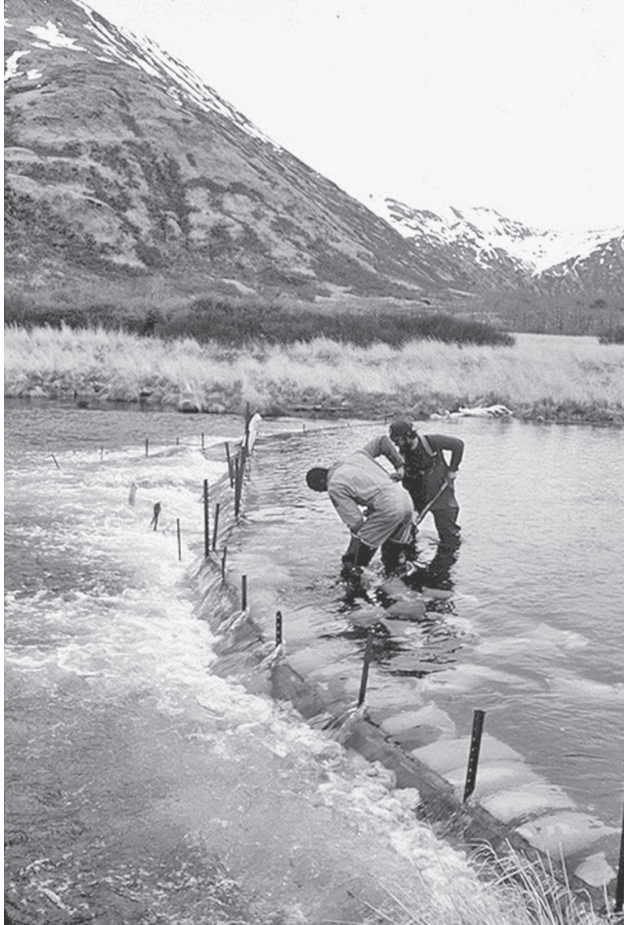
Barrier placed in the O'Malley River to stop the upstream migration of sticklebacks into O'Malley Lake, 1985-87. (Jim Finn, Anchorage, AK)
