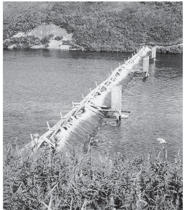
Karluk River salmon counting weir at the Portage, 1944. (Jerrold M. Olson, Auke Bay, AK)
