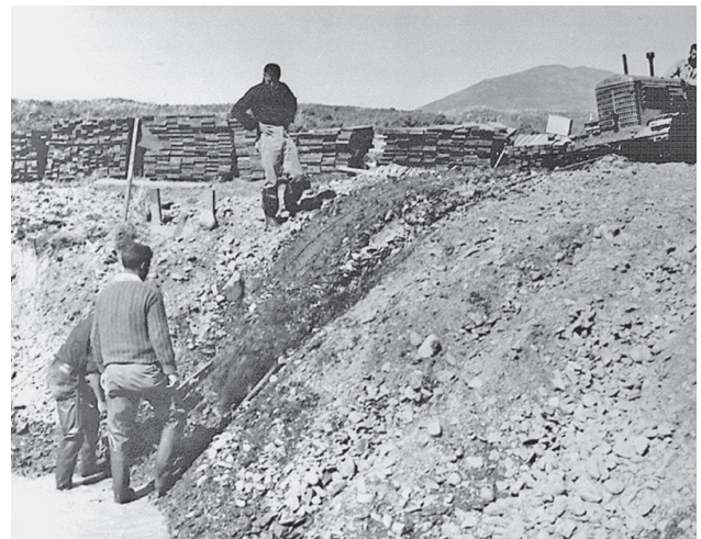
Excavating footing for a two-way weir, upper Karluk River, June 1949. (Richard F. Shuman, Auke Bay Laboratory, Auke Bay, AK)
