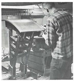
Model of radial gate used in the Tarbela Dam.
