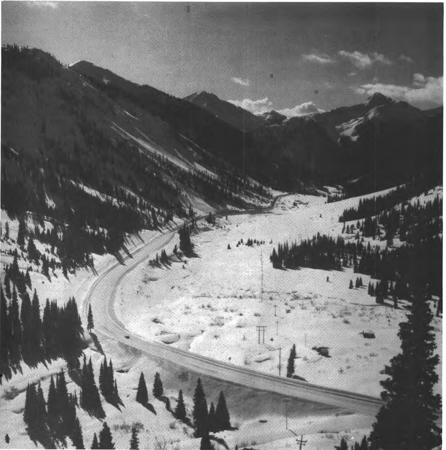
Plate 1. The view south along Highway 550 from below Red Mountain Pass. The Brooklyns avalanche paths threaten the highway from the east (left). From the opposite side several major paths, including Imogene, Bismark, and Battleship, cross the highway and damage timber on the reverse slope when they run full-track.
