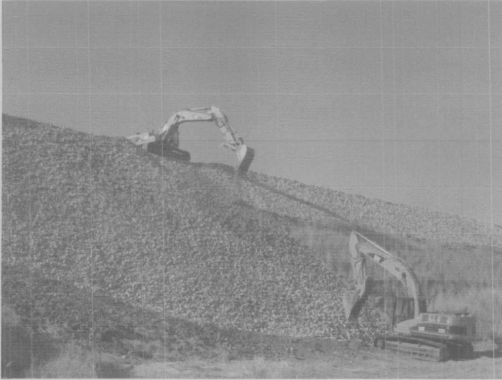
Photograph No. 2-3. Tooele Valley Railroad Grade, Extension Section
