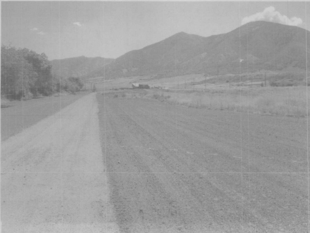
Photograph No. 2-4. Tooele Valley Railroad Grade, School Section
