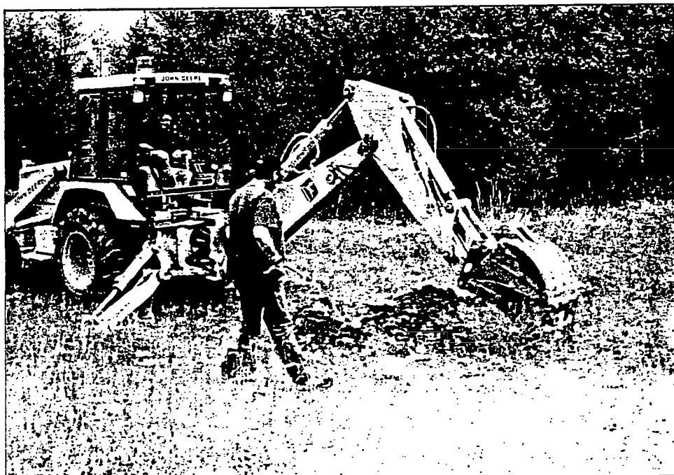
Figure 42. Site 3 - Excavation of TP-6.
