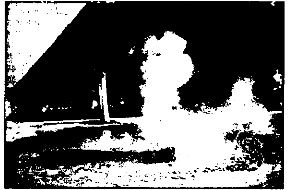
Vents evolve steam as Geo-Cleanse destroys xylenes and phthalates in ground water.
