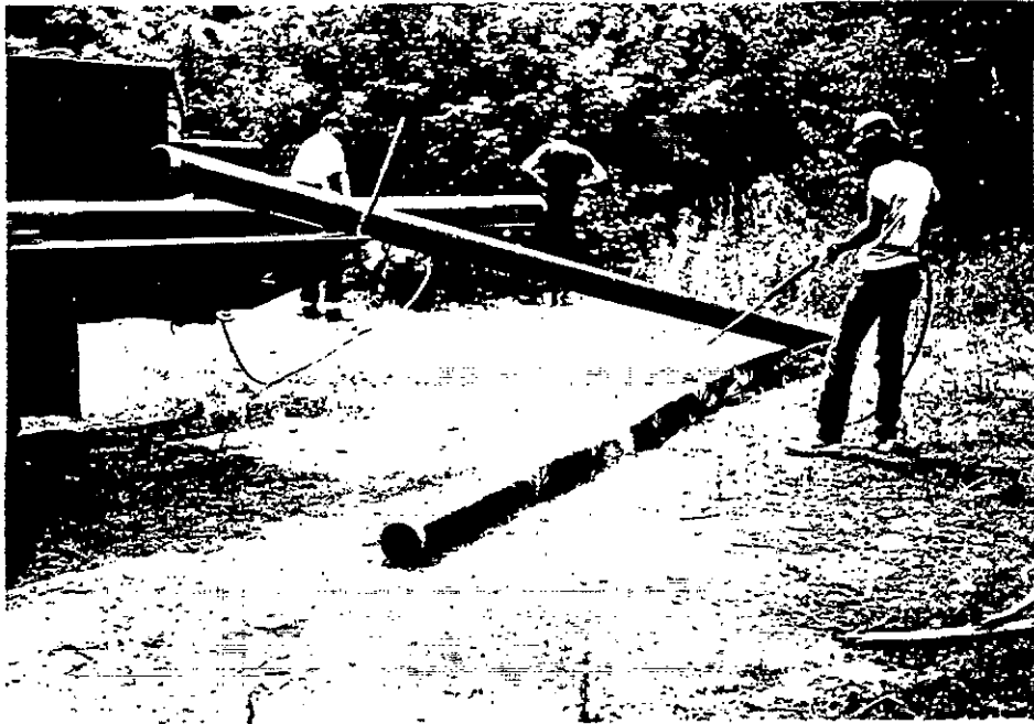
— Photo 3 — — Houston Taylor steam cleaning outside of — — casing. —
