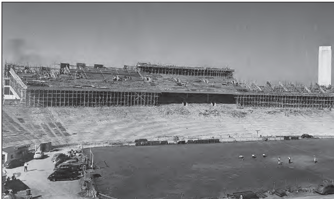
1948: Cotton Bowl Stadium - known far and wide as "The House That Doak Built" - received a facelift in the late 1940s with the addition of upper decks on both sides of the stadium. To satisfy the growing demand to watch Doak Walker, SMU's great All-America halfback and Heisman Trophy winner, a total of 21,231 seats and a new press box for the nation's media were added in 1948. When work was completed a year later in 1949, capacity rose to 75,504.
