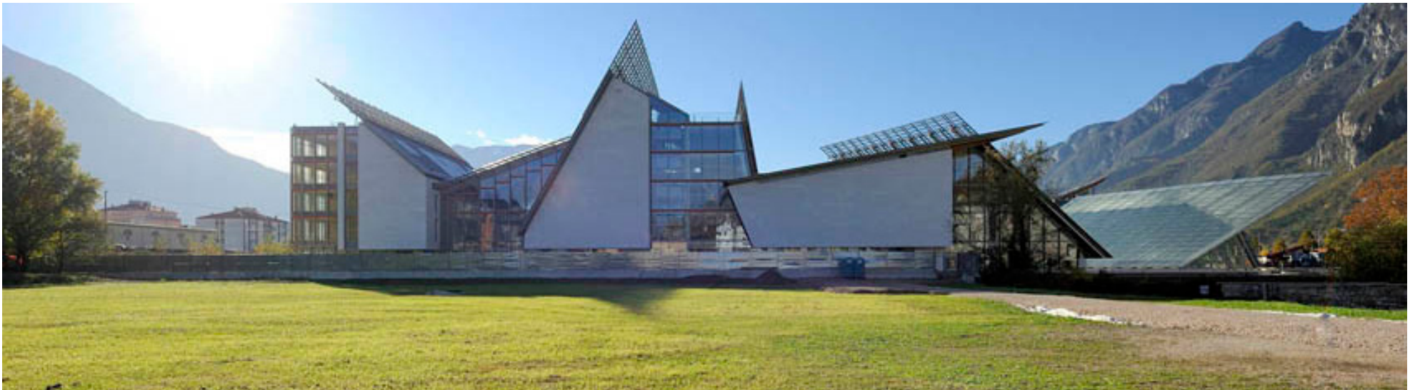
3.11_ Photo of the finished building ( http://www.archdaily.com/423101/muse-renzo-piano/522136ffe8e44e711f00001e-muse-renzo-piano-photo )
