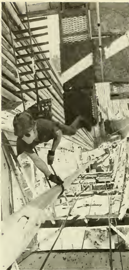
A derrick or "monkey" man works high above the drilling platform. Photo by David Moody © 1978.
