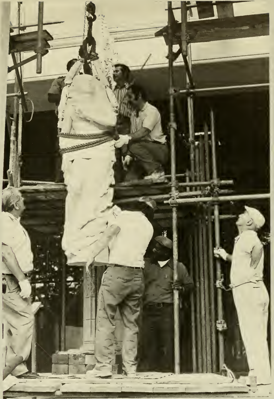
White-gloved stone carvers Frank Zic, Vincenzo Palumbo, and Roger Morigi and members of the building crew carefully hoist the completed stone carving of Adam to its rightful niche outside the Cathedral's West Front. Photo by Morton Broffman © 1978.
