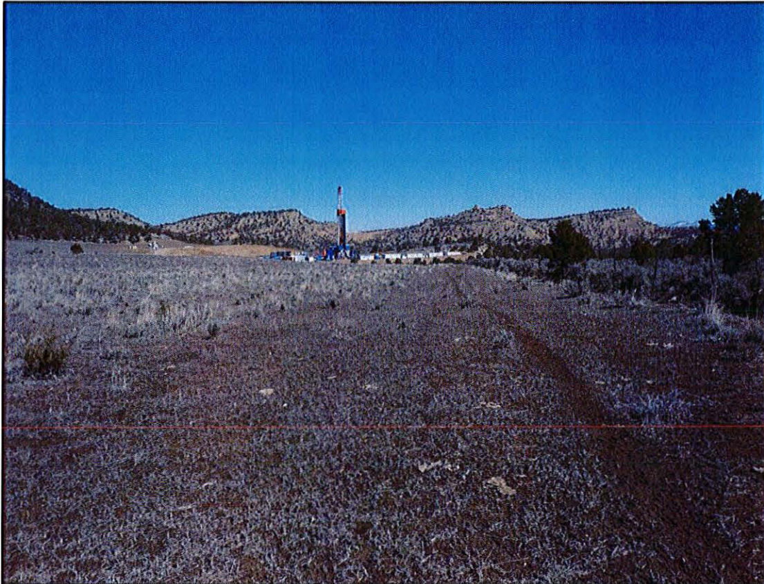
Cover Photo: Looking north toward O19EB along proposed pipeline alignment.
