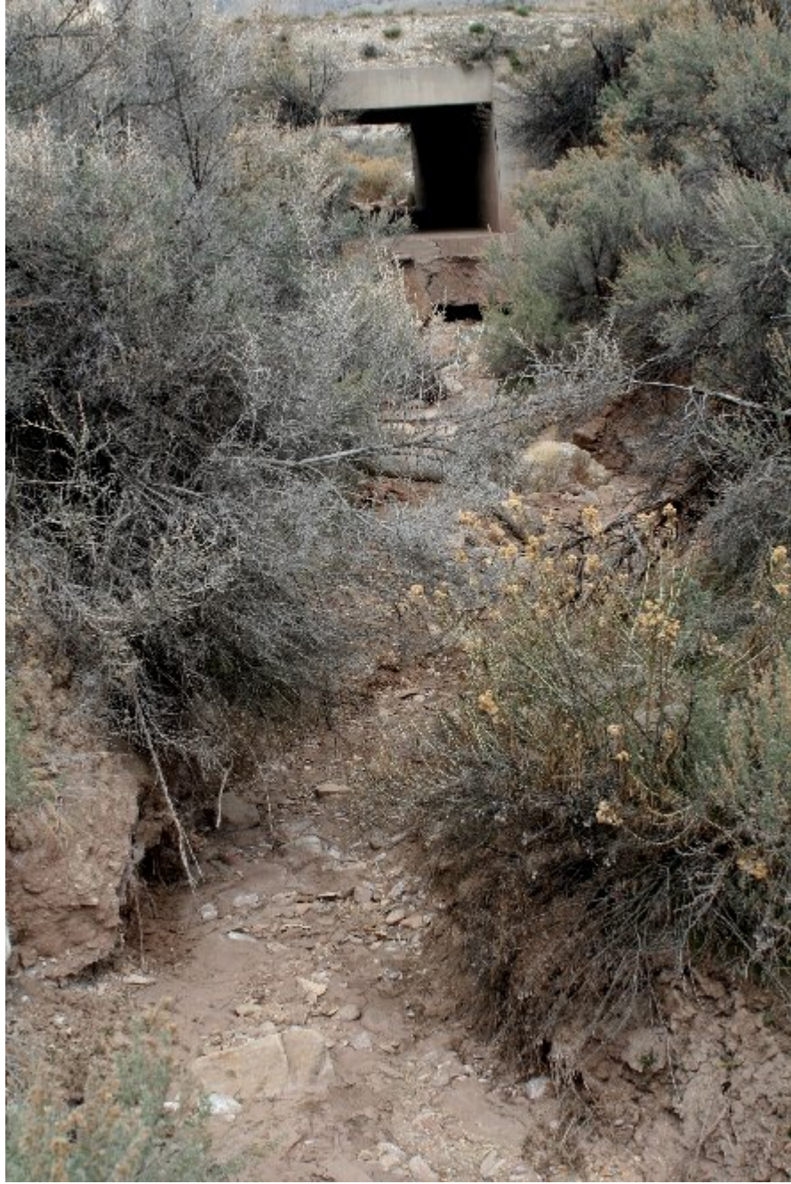
Photo 4. View north through second box culvert on the 20 acre parcel.
