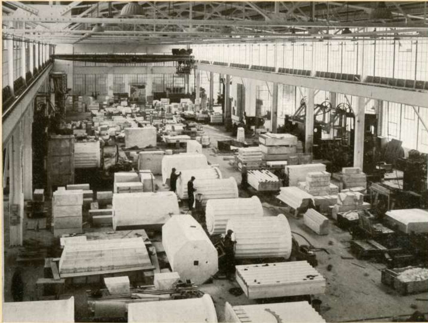
Exterior Building Shop, Proctor, Vt., with column drums for United States Supreme Court Building in foreground
