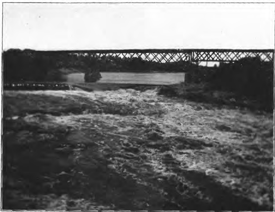
B. DAM AT BLACK RIVER FALLS, WIS., PARTLY CARRIED AWAY BY HIGH WATER.
