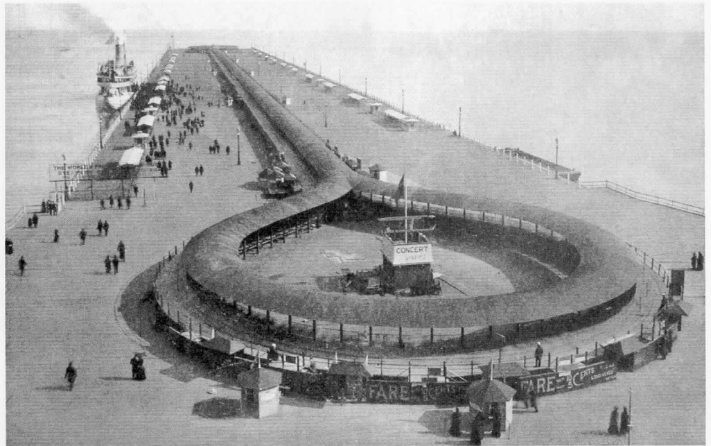
Figure 17. A moving sidewalk made a complete circuit of the 2500-foot-long pier that extended into Lake Michigan.
