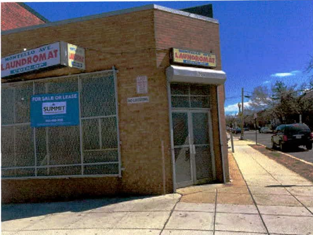
1. Front of subject property, view from west
