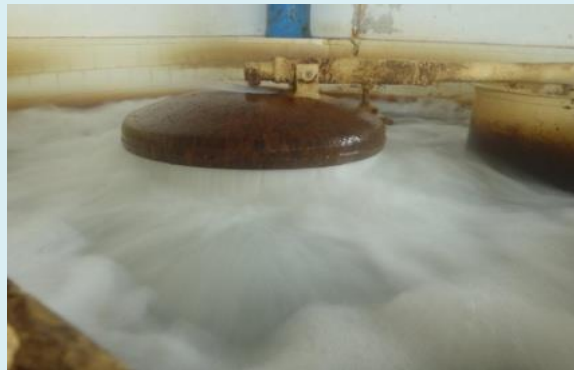
Figure 37 Water pressure dissipation using a load breaker
