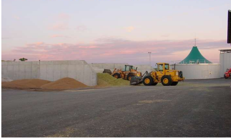
Maize silos, digester and gas storage of the Energy Crop Digestion Plant Reidling
