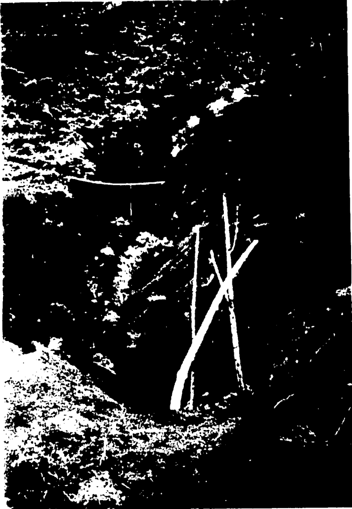
Photo 22: These PVC pipe spans are in the pipeline serving the village of Cayara, Potosi. Such exposed spans should always use galvanized steel pipe, but the project had to substitute plastic pipe temporarily because of a long delay in the delivery of the steel pipe which will later replace it. Many of the systems faced this management problem during construction.
