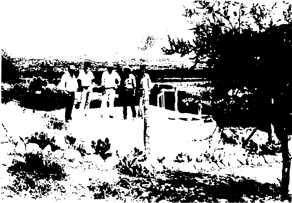
Photo 16: This water storage tank in the village of Chalarmarca, Tarija, is typical of tanks constructed by the project. It is well designed and solidly constructed.
