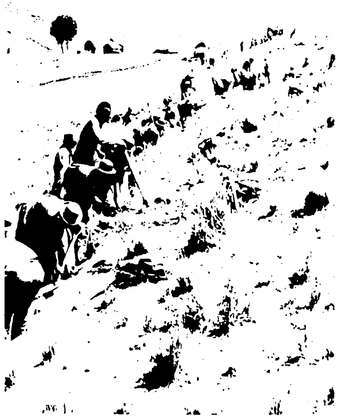
Photo 6: The whole community, women as well as men, has turned out in Ajlla Pata Pata, La Paz, to work on construction of their long-awaited water system. Construction was delayed nearly three years while this community worked out an agreement to share a water source with another community.
