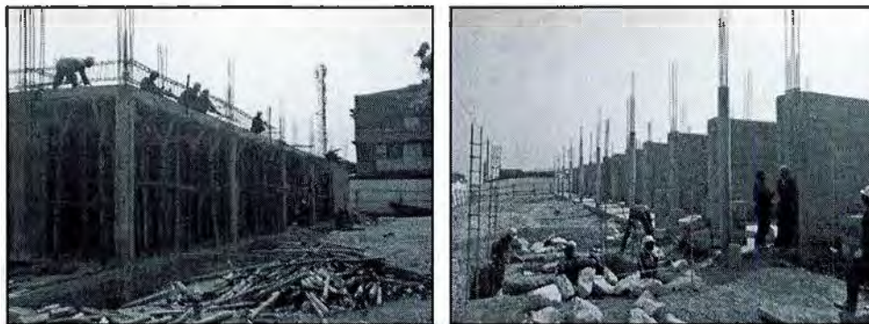
Arua taxi park under construction
