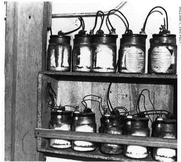
Acid-filled, wet-cell batteries, such as this group of ten, powered turn-of-the-century electric actions.
