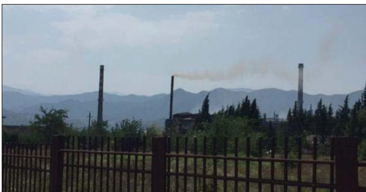
Figure E-2: Visible Air Emissions from GAA Plant, 2017 (taken from boundary of the Project road around KM 11.1)
