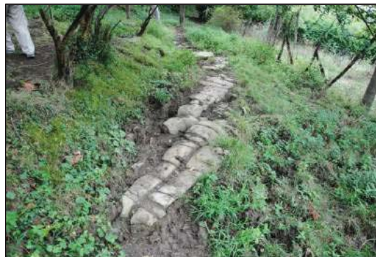
Figure E-41: Stonework in Zestafoni
