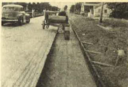
FIG. 9.—Rolling base course in widened trench with trench roller.
