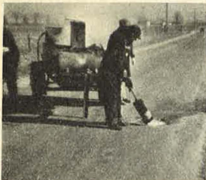
FIG. 5.—Winter patching—drying damp hole preparatory to filling with bituminous mixture.
