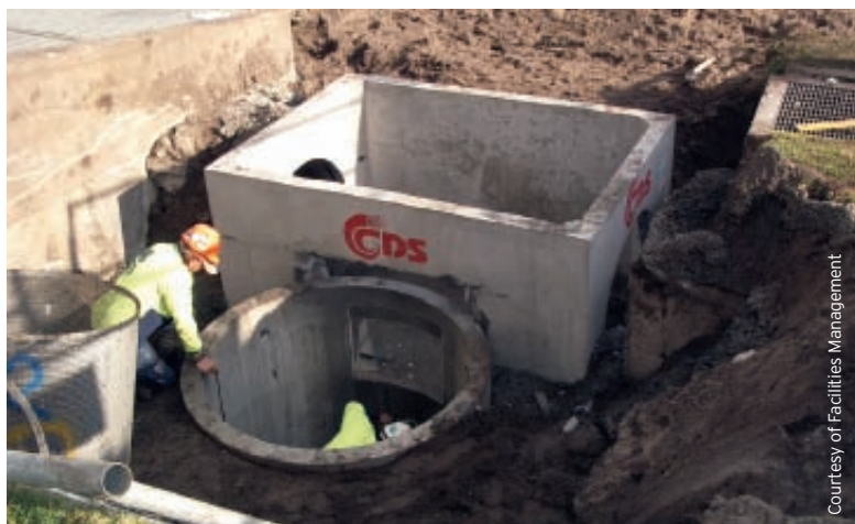
Constructing the University's percolation pit.
