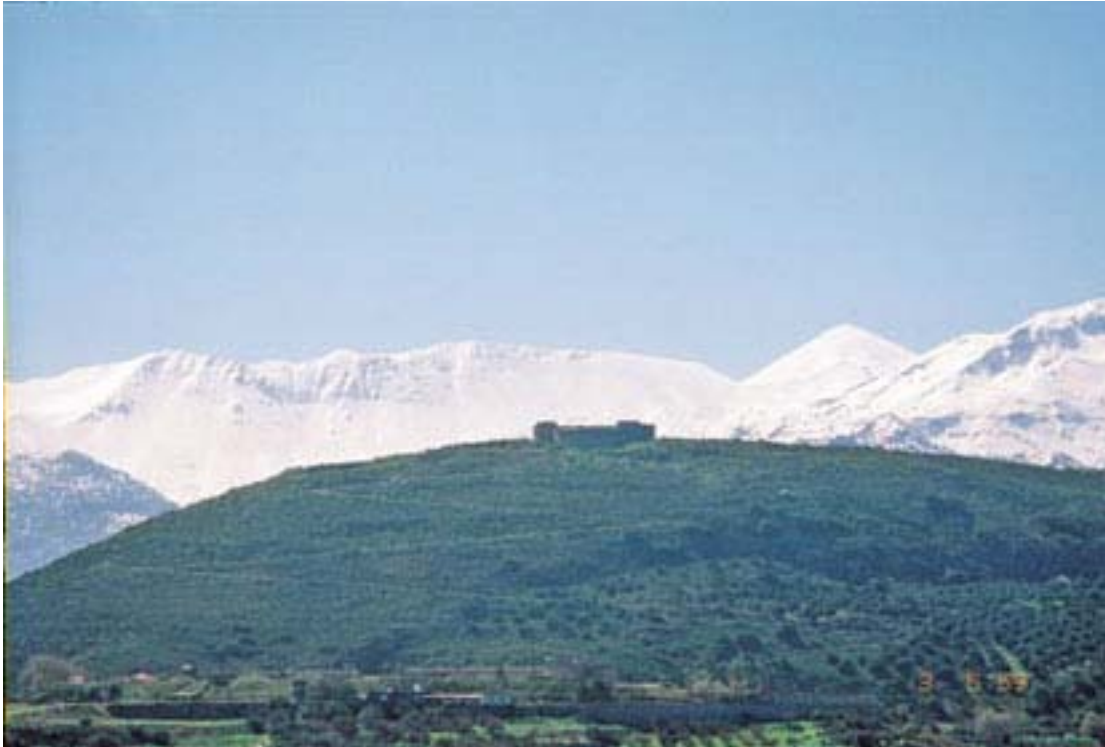
Akra Soudha—Abandoned fort from N
