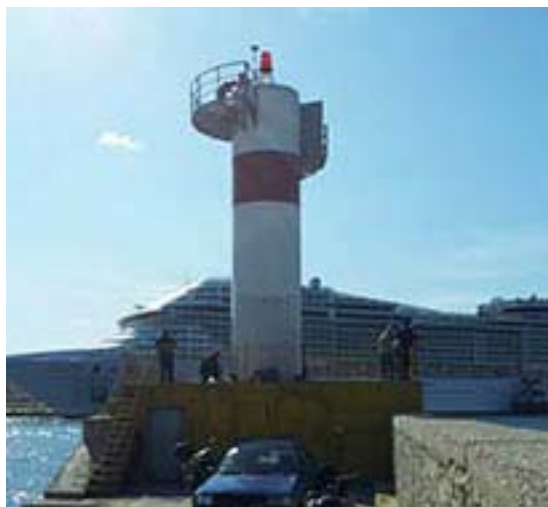
Molos Vasileus Yeoryios (ight at head of breakwater)
