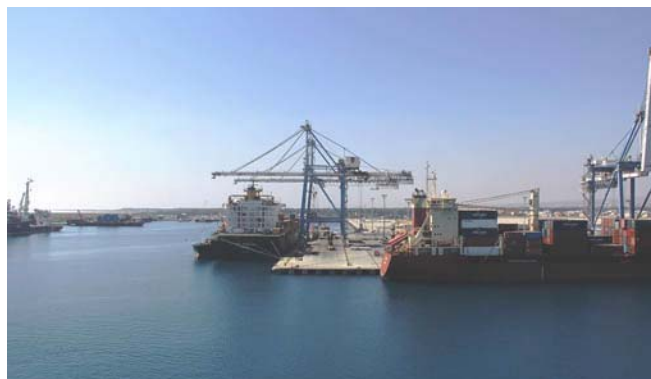
Limassol Container Terminal
