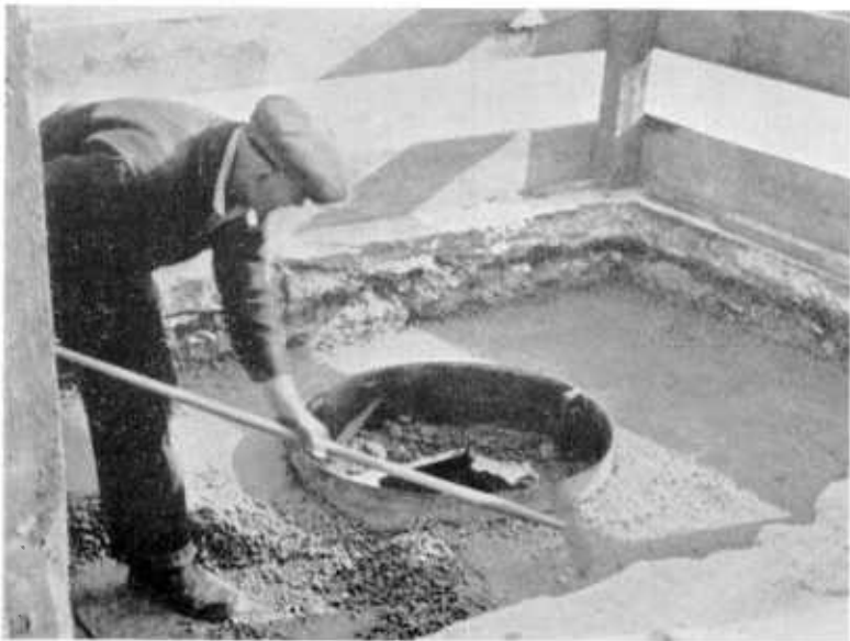
PATTERSON PARK AVENUE AND MONUMENT STREET POURING ROOF OF MANHOLE
