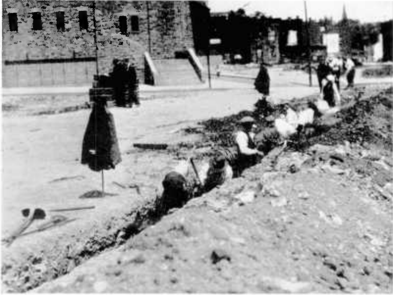
HOWARD STREET EXTENSION PROJECT. MAKING LATERAL CONNECTIONS (P.W.A.)
