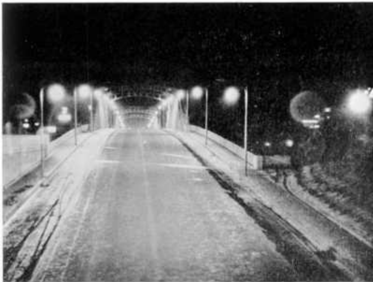
HOWARD STREET VIADUCT LOOKING NORTH (NIGHT VIEW)
