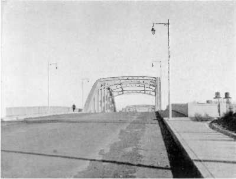
G. E. TYPE 81D LUMENAIRES ON THE HOWARD STREET VIADUCT
