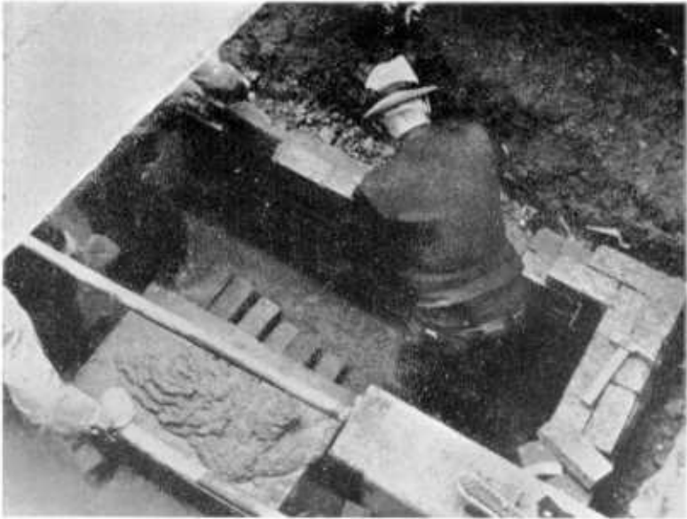
PATTERSON PARK AVENUE AND MONUMENT STREET BUILDING BRICK MANHOLE
