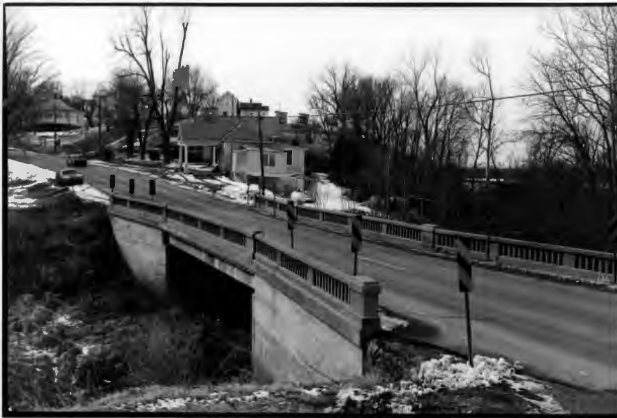
This concrete bridge over Hicklin Branch is at the east end of Napoleon, Lafayette County's westernmost city which was platted originally as Lisbon in 1836.
