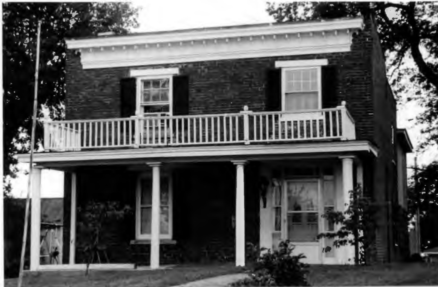
Councilman House 1858-59 (1988 photo)
