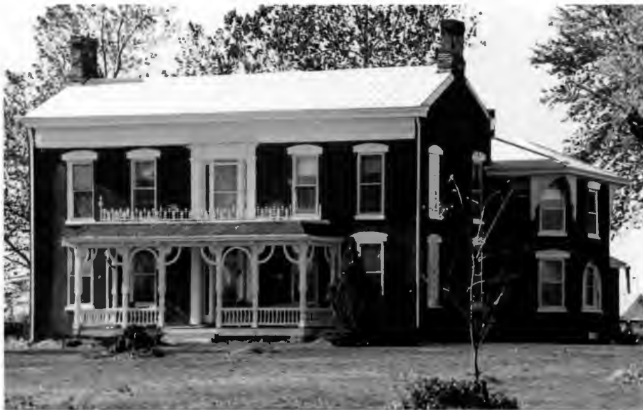
Shields House ca. 1850s (1988 photo)
