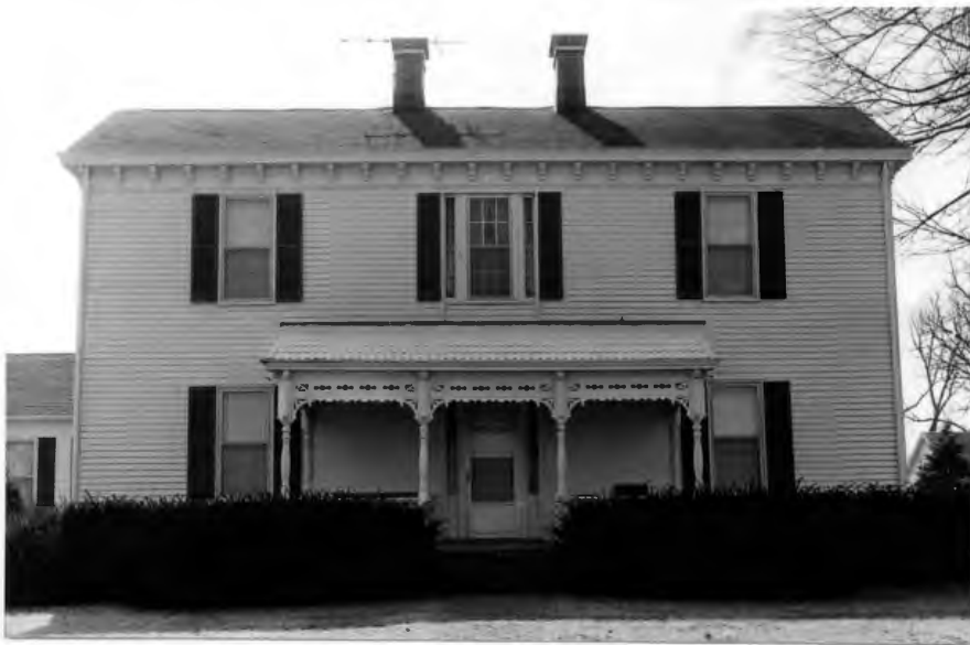
Barnett-Slusher House 1868-69 (1989 photo)
