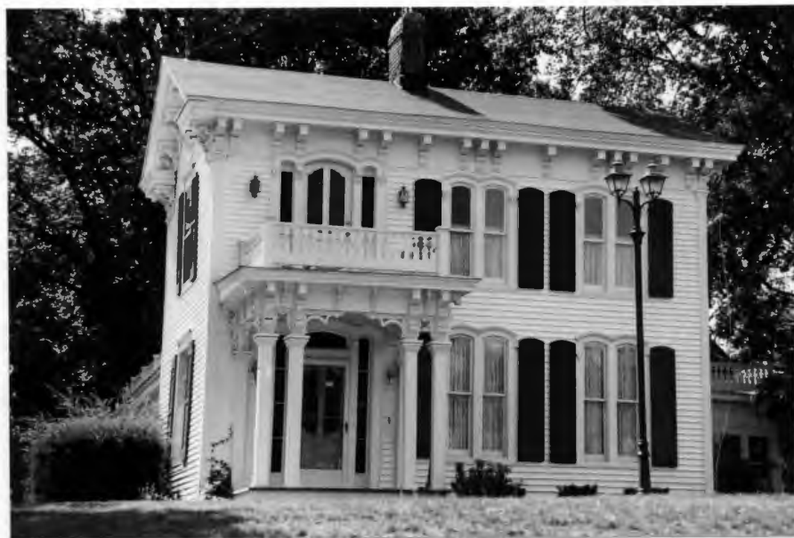
Corder-Brown House ca. 1870; 1900 (1988 photo)
