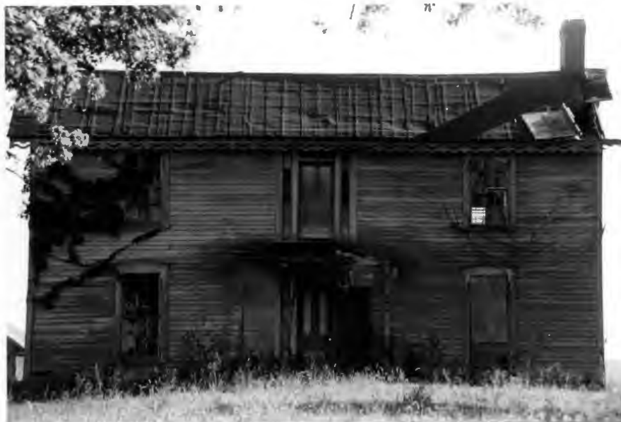
Spencer W. Brown House ca. 1850s (1988 photo)
