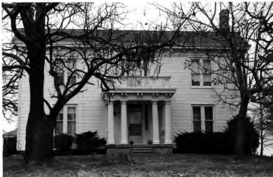
Andrew Jackson Slusher House 1851/1869 (1988 photo)
