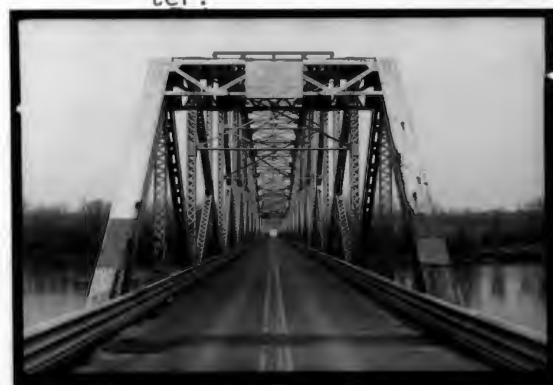
Waverly Bridge looking north
