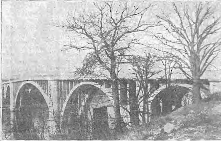
Cappelen Bridge, Minneapolis.
