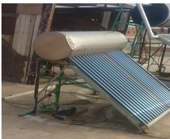
Fig. 1. Evacuated tube solar collector
