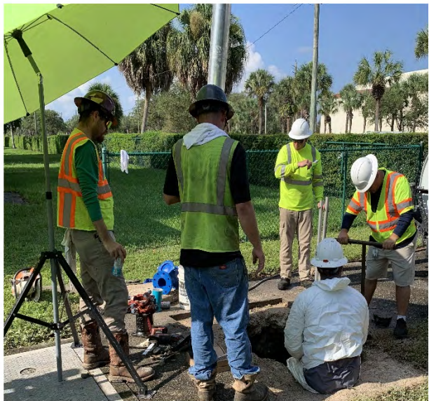
At left: Construction employees Tommy Cox and Wyatt Fischbach replace a valve in LS152. The space does not meet the criteria for an official “Confined Space” entry nor did it require shoring safeguards due to limited depth of the hole, but this activity is certainly performed in a cramped environment as Tommy entered the work zone to assist Wyatt on this very hot day. Both men are utilizing appropriate PPE while Wyatt is wearing the white Tyvek coveralls. A sheet of plastic is used as a barrier to prevent any inadvertent leakage from contacting the soil.
