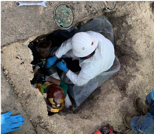
At Right: Construction employees Robbie Spires, Tommy Cox and Wyatt Fischbach are working together with Jerry Suarez-Prado, Collections Systems Forman, and Kyle Shepherd to support the valve replacement. Collections was supporting this activity by initiating lockout / tagout on the LS 152 electrical panel and closing the valve upstream of the work zone. Industrial umbrellas are being used regularly during these very hot days to prevent heat stress. Plenty of fluids were available and consumed during this task.
