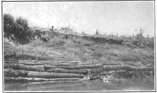
Timber toedam to prevent undercutting of levee.
