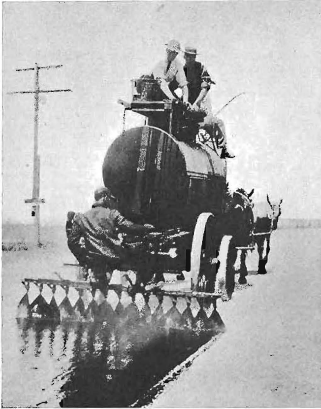
Horse-drawn equipment spreading asphaltic oil surface on concrete pavement north of Fresno in 1913. Modern asphalt spreader.
