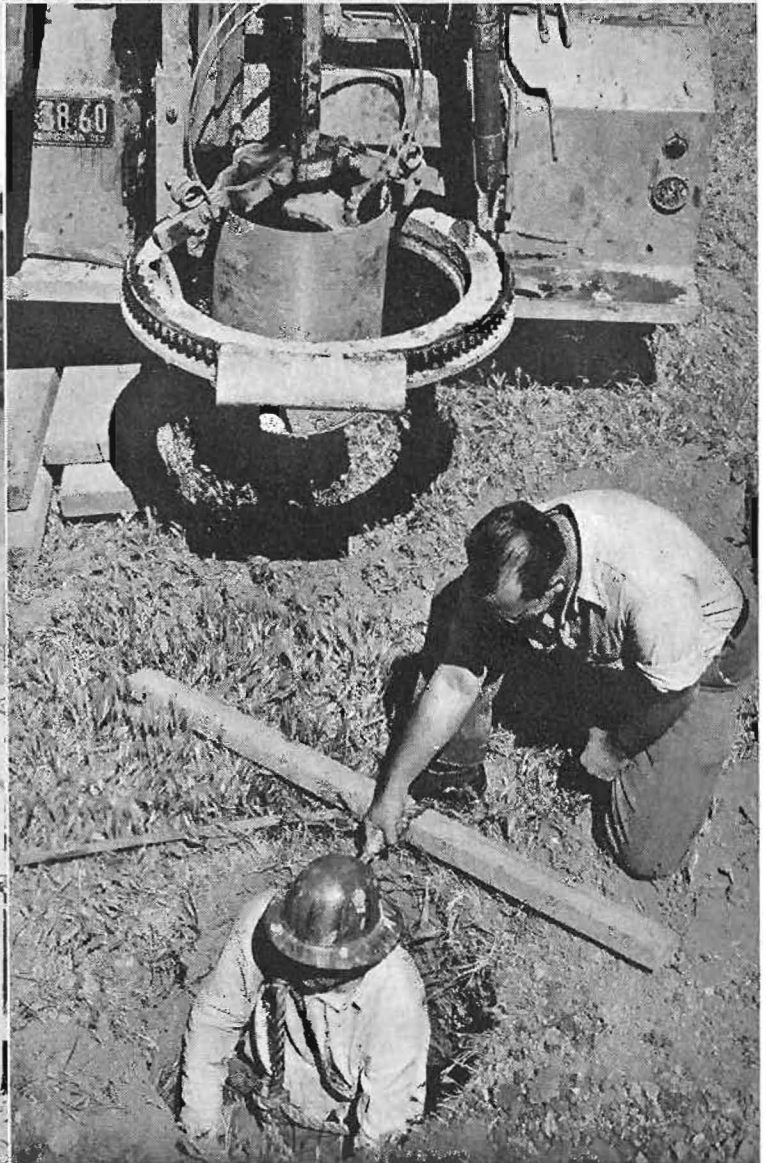
Upper—Combination foundation drilling equipment dismantled and ready for road. Lower left—Closeup view of rig showing sand bailer, extension rod for soil sampler, churn bit, rotary bucket with Kelly bar and driving yolk, and the sampler assembly. Lower right—Foundation Inspector sitting in top of 30-foot boring following inspection of the ground to bottom of an 80-foot hole.
