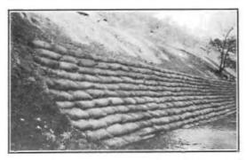
Sacked concrete riprap protecting embankment of newly constructed 24-foot graded roadbed in Lake County, a portion of the Ukiah-Tahoe state highway.
