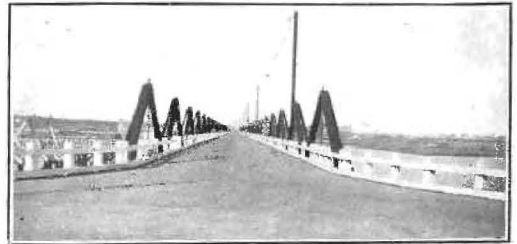
View of Rio Vista Bridge.
