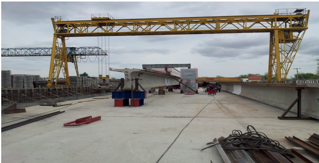
Figure 16 General view of the power stand and the VTK-33u tested beam
