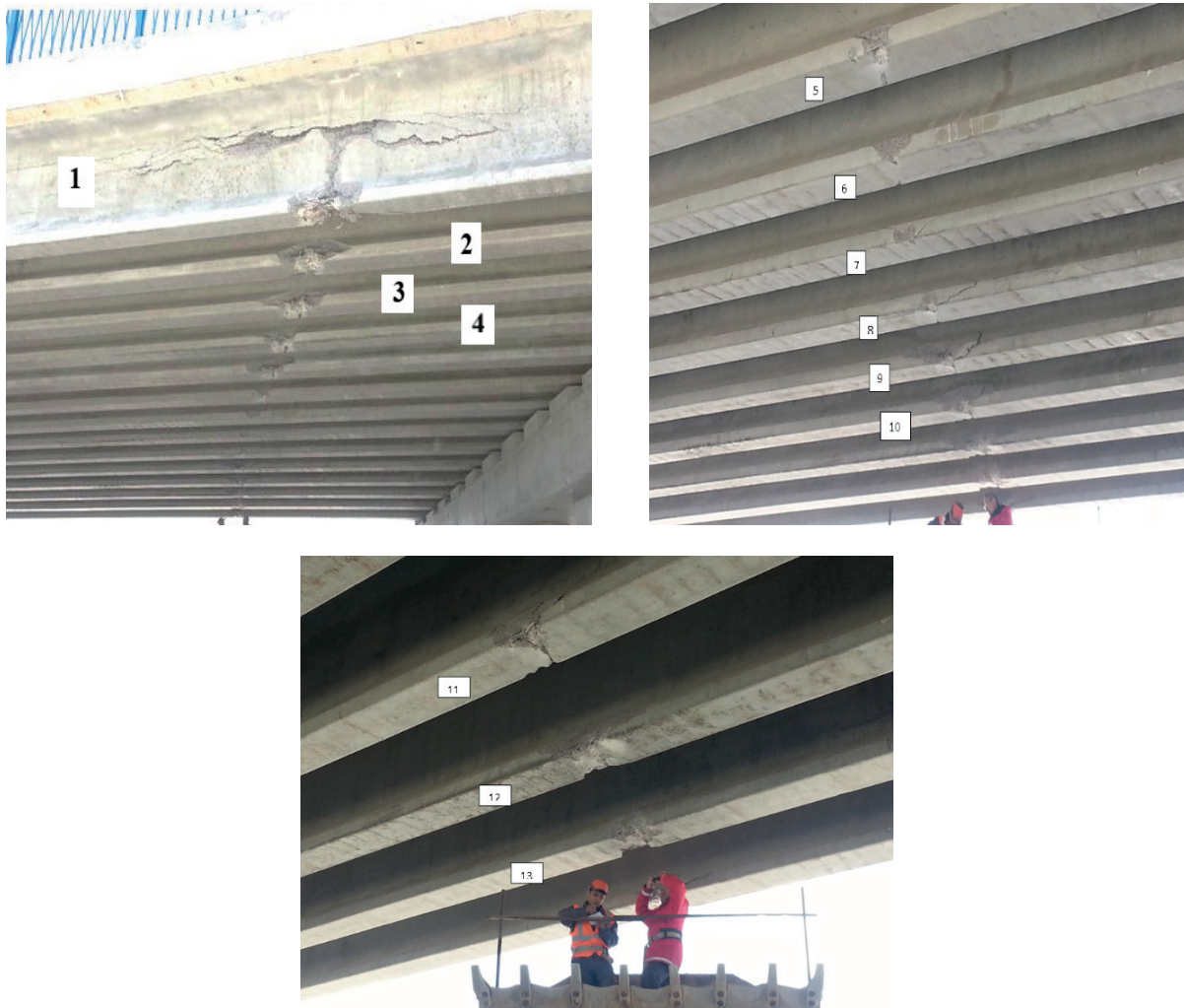
Figure 2 The general view of the damaged superstructure No. 1 from the Kapshagai city side
