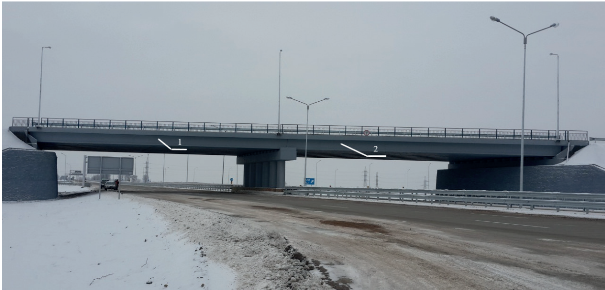
Figure 1 The general view of the overpass from the Kapshagai city side: 1 and 2 - superstructure numbers
