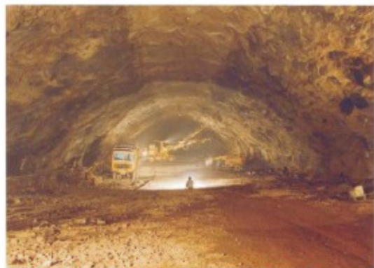
Machine Hall Cavern, Ghatghar H.E. Project, Maharashtra, India
