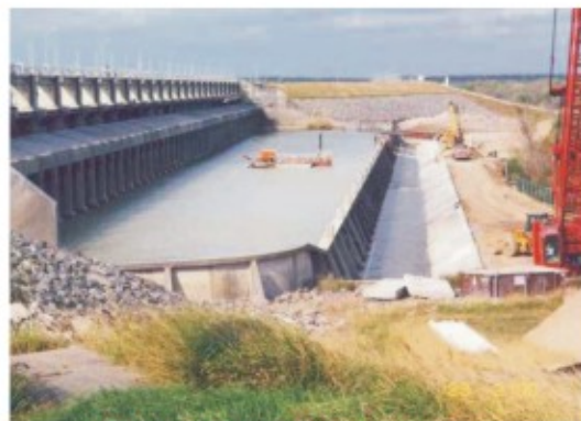
Filling Hearth Floor of Dam in Spillway (USA)
