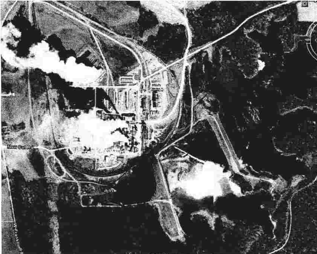
Figure 2-1 Aerial View of A.B. Brown Station
