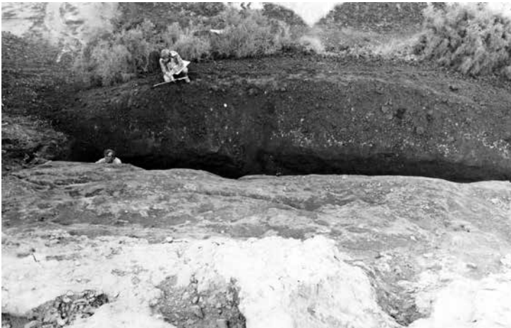
Figure 5.32. Section cleaning from above.
