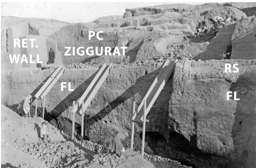
Figure 5.25. Watelin's demolition of the Retaining Wall to expose the face of the larger ziggurat; red stratum and flood level are indicated (FM 74538).
