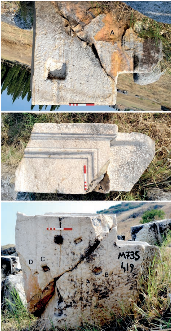
8. - Stoa-basilica, central sector, upper part of a pillar: metal cramps (B-D) were used to secure the block, along the fissure produced by a travertine inclusion (A).
