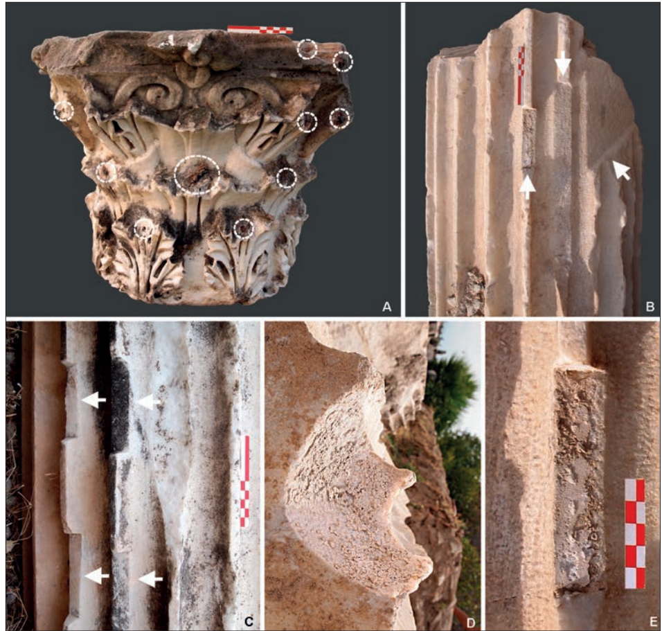
11. - Sanctuary of Apollo, Corinthian upper portico: replacement parts were used to restore damaged flutes, leaves and volutes.
