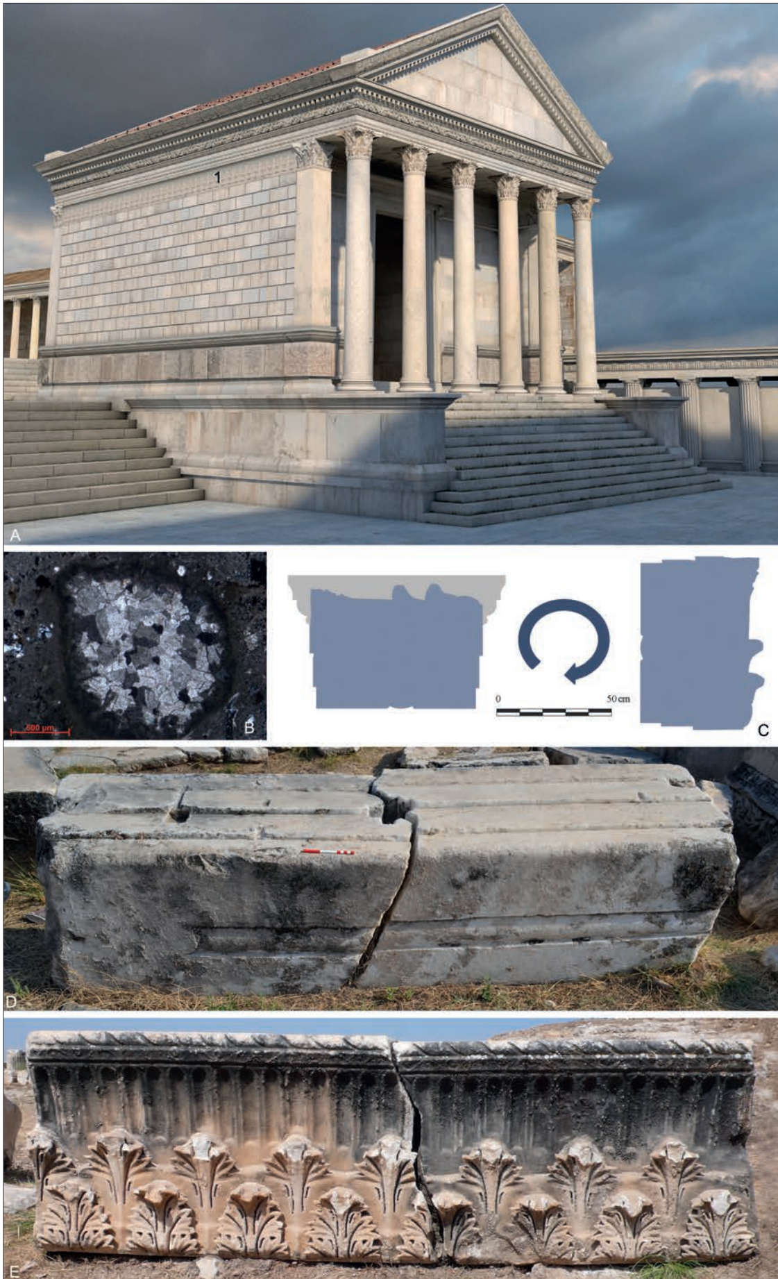
16. - Sanctuary of Apollo, Temple A: reconstruction of the Severan building (A, by M. Limoncelli); B: thin section showing a marble fragment only partially burnt inside the mortar; C: the architrave of Temple B was sculpted only on the upper face and rotated to obtain a fluted wall frieze; D-E: Ionic architrave of Temple B reused as a fluted wall frieze.
