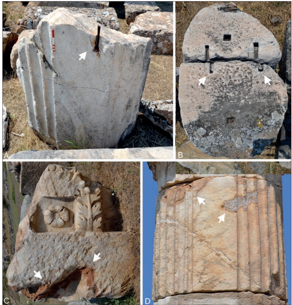
9. - Stoa-basilica, A: Ionic stoa, double half-column restored with a metal cramp on the side; B: Ionic stoa, double half-column restored using two cramps on the bottom face; C: central sector, cornice showing a travertine vein along the inner face; D: Ionic stoa, double half-column drum showing imperfections and a travertine vein.
