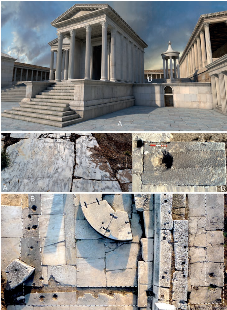
4. - Sanctuary of Apollo: the pavement slabs of veined marble from Denizli (A) enhance the white walls of Temple A; grey slabs of Marmar Tepe quality support a metal fence around the oracular Monopteros, visually marking the boundaries of this sacred area.
