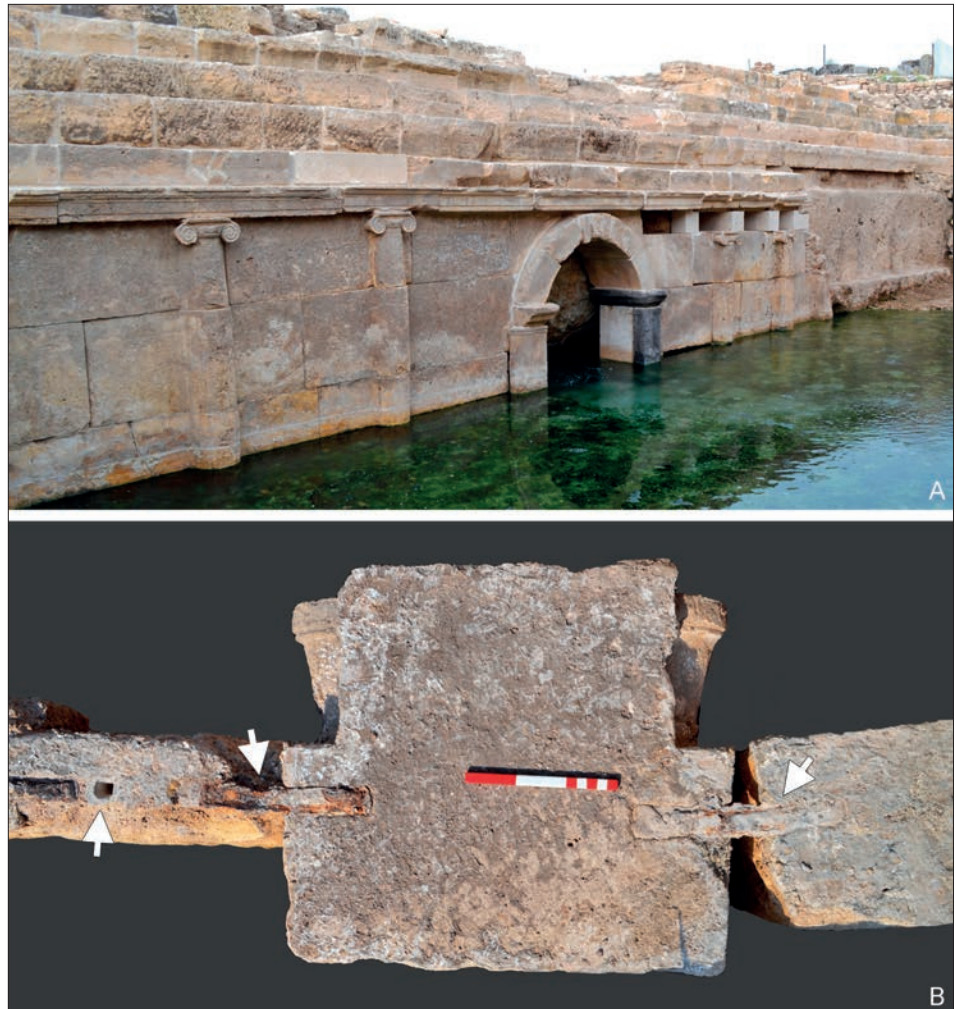
17. - Ploutonion: the Ionic façade in front of the sacred cave (A); the upper faces of an Ionic capital and the adjacent wall slabs, with iron cramps in situ and a dowel hole (B).
