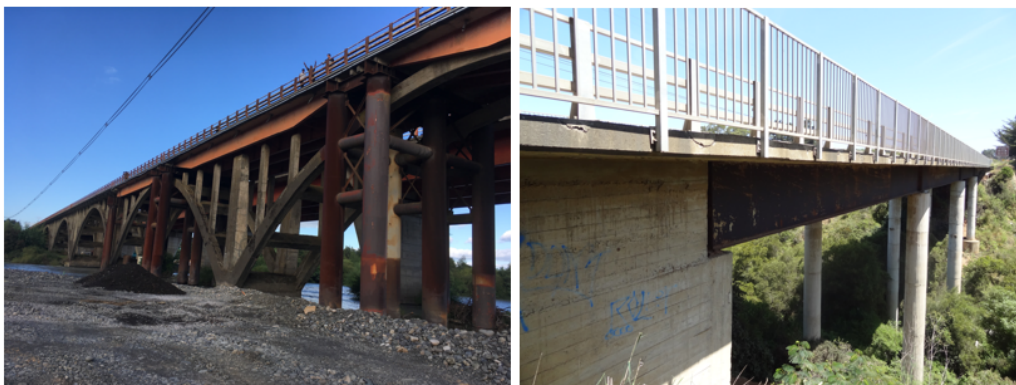
Figure 1: Tolten bridge (left) and Seminario bridge (right).
