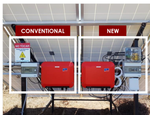
Figure 6: Installation of the system.
