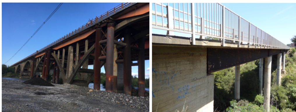
Figure 1: Tolten bridge (left) and Seminario bridge (right).
