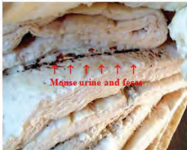
Figure 2. Mouse urine and feces on insulation.
